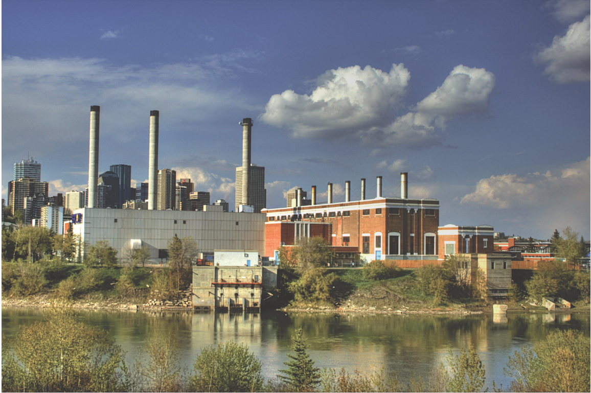
Figure 80. Buildings of the Rosedale Power Plant in Edmonton, Alberta. WinterforceMedia, 2010.
