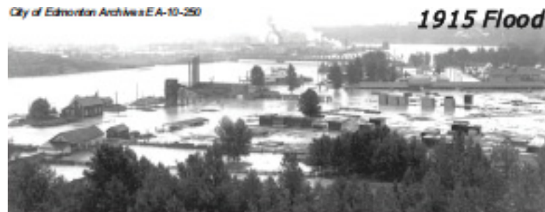
Figure 29. 1915 Edmonton Flood. From Geoscape Edmonton.
