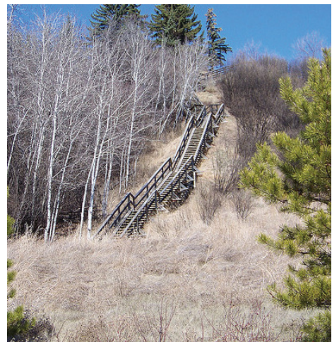
Figure 48. Photograph of Wood Stairs, Edmonton river valley. 2010.
