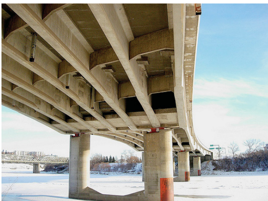
Figure 76. Photograph Underneath Bridge
