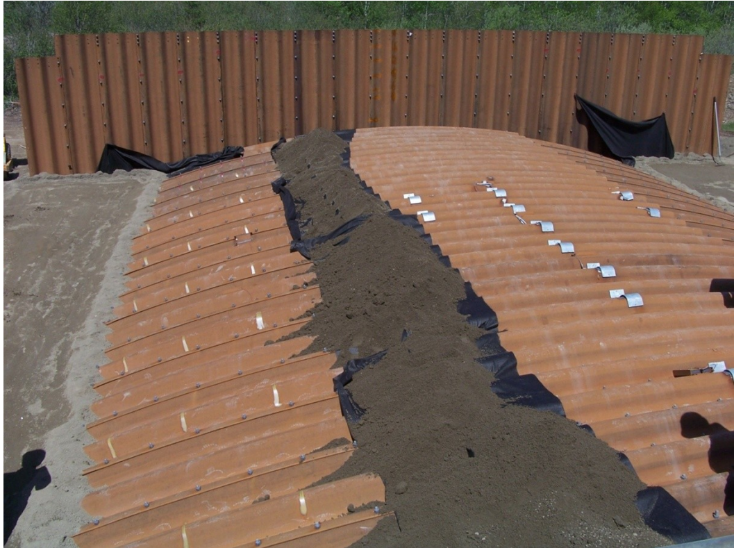
Figure 4-2 – Partially Buried Test Structure
