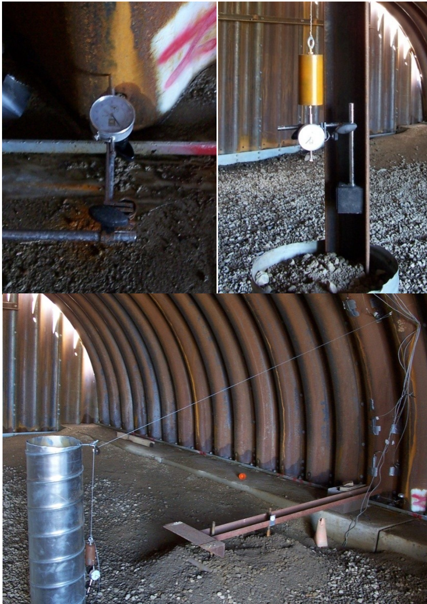
Figure 4-13 – Manual deflection gauges at the footing, crown, and haunch
