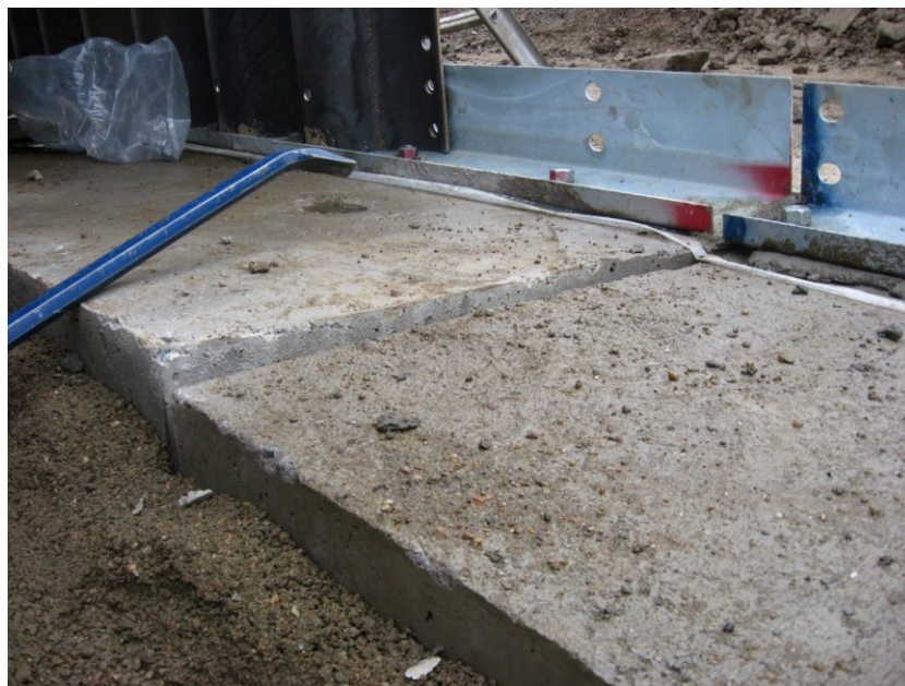
Figure 4-6 – Precast Footings
