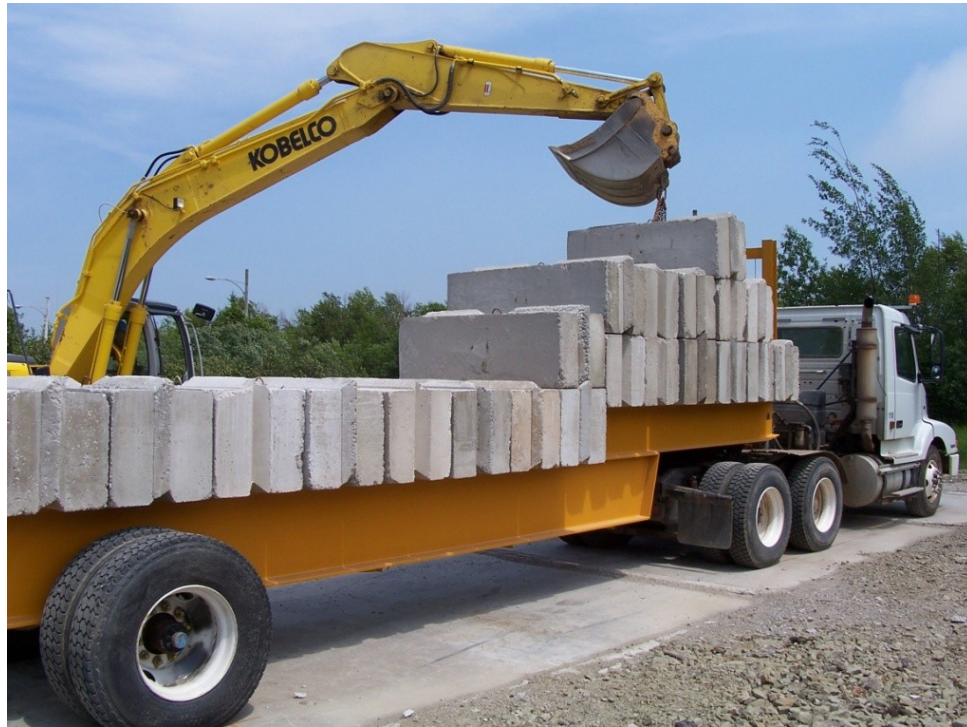
Figure 4-18 – Test frame during loading
