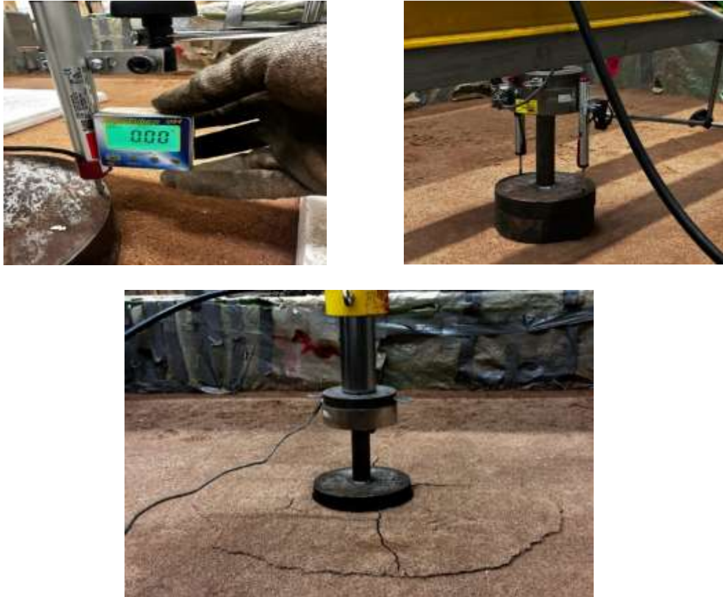
Figure 3.12: Plate Load Test Setup
