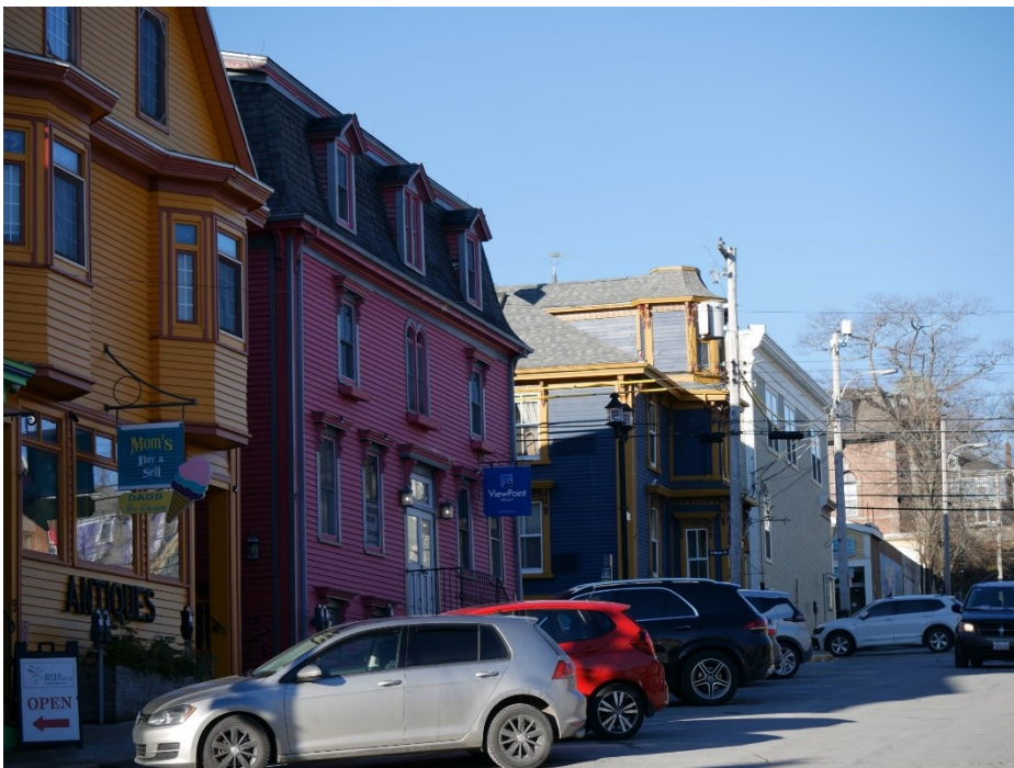
Buildings Within Commercial Zone 1 on South End of King Street
