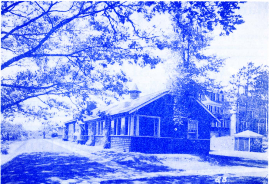
Summertime at the San. Pavilion 1 with West Infirmary in background.
