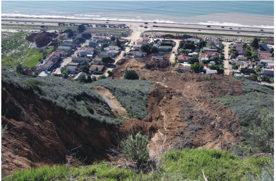
Figure 12 View from the main scarp down the length of 2005 landslide [84].
