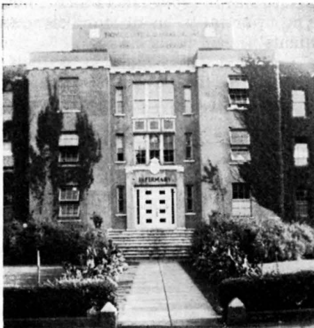
Former Entrance, East Infirmary
