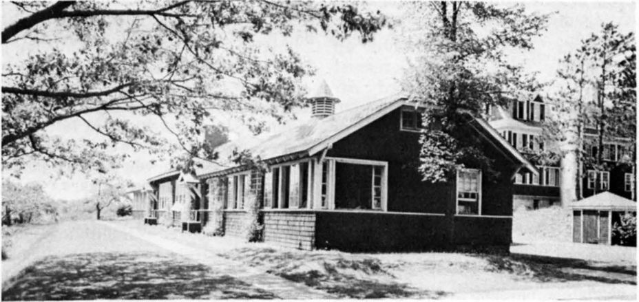
Pavilion 1, with West (Old) Infirmary in background
