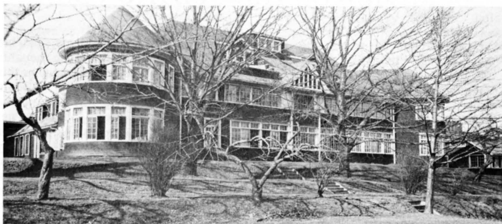
The original Provincial Sanatorium, built in 1904; later remodelled and used as the Women's Annex.
