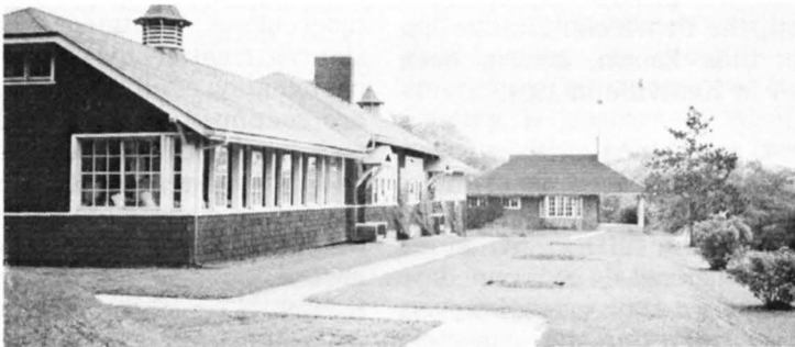
Pavilion 2 and Library
