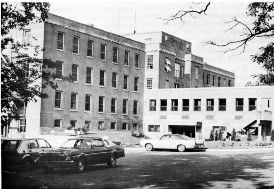
East Infirmary from north-east, showing new Service Building, with new entrance. Administrative offices, admitting office, reception desk, waiting room, canteen and stores departments on the lower level. Cafeteria and dietary department on upper level.
