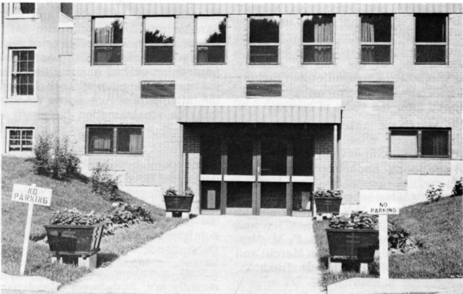
New main entrance to Miller Hospital, east side of service building.
