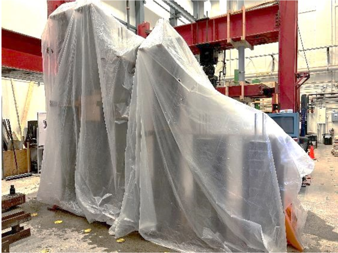
Figure 3.6. Curing of columns using water spray and plastic coverings.
