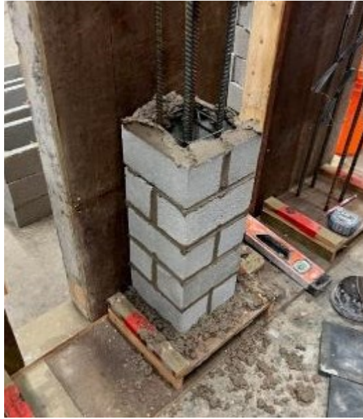
(a) Before Grouting (C-shaped)
