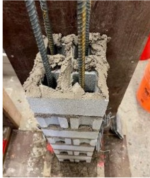
(b) Before Grouting (Stretcher)
