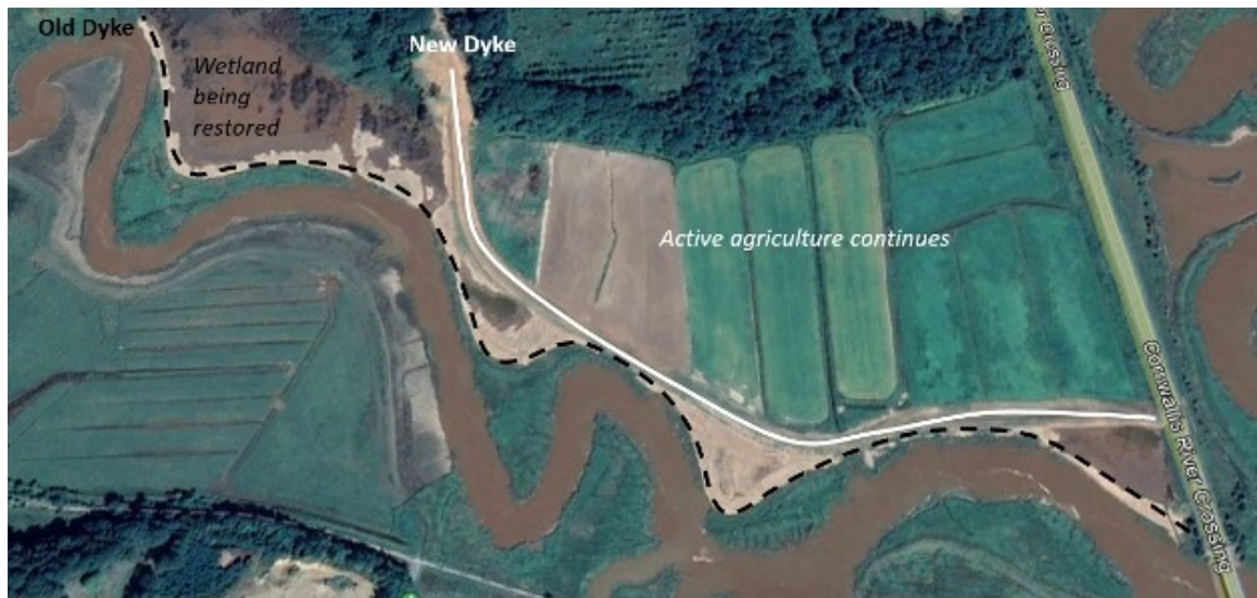
Figure 5: Managed Dyke Realignment project at Belcher Street Marsh in Kentville, Nova Scotia along the Jijuktu'kwejk (Cornwallis) river. The old dyke which followed the coastline when it was built was realigned to a more linear dyke protecting only active agricultural land and allowing restoration of foreshore tidal wetlands. Created by Kate Sherren using Google Maps imagery.
