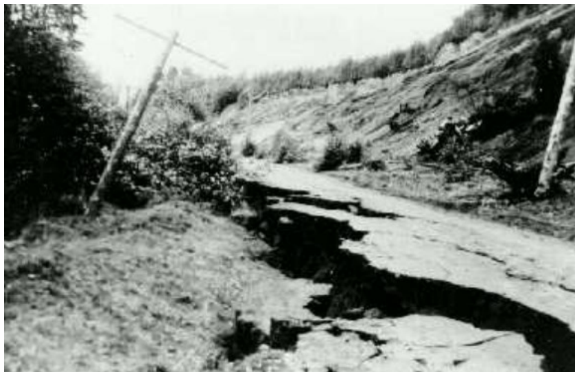
Figure 2. Kelsey Bay highway after the 1946 earthquake
