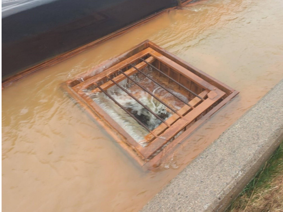
Figure A.11 Overflow weir to natural wetlands with high flow in channel between settling pond and constructed wetland for System 1.
