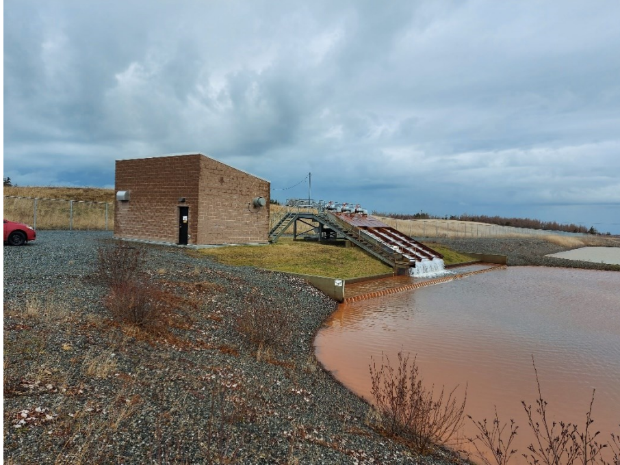
Figure A.3 Caustic building and aeration cascade at settling pond inlet for System 2.
