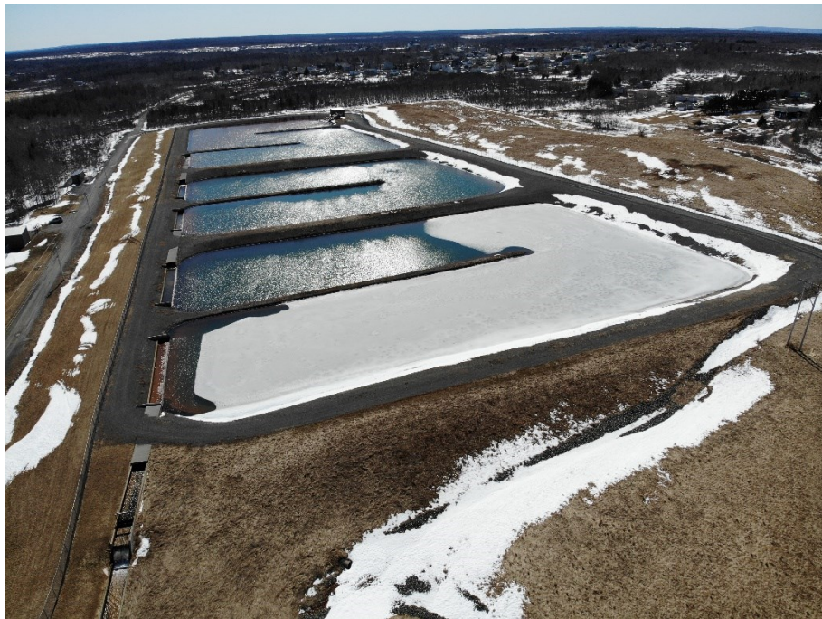
Figure A.6 Three settling ponds for System 2.
