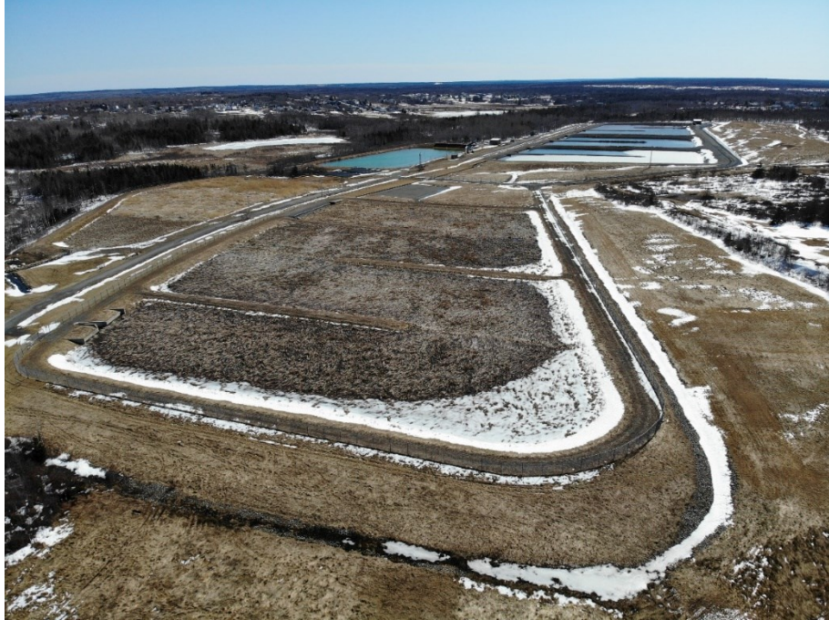
Figure A.15 Constructed wetland for System 2.
