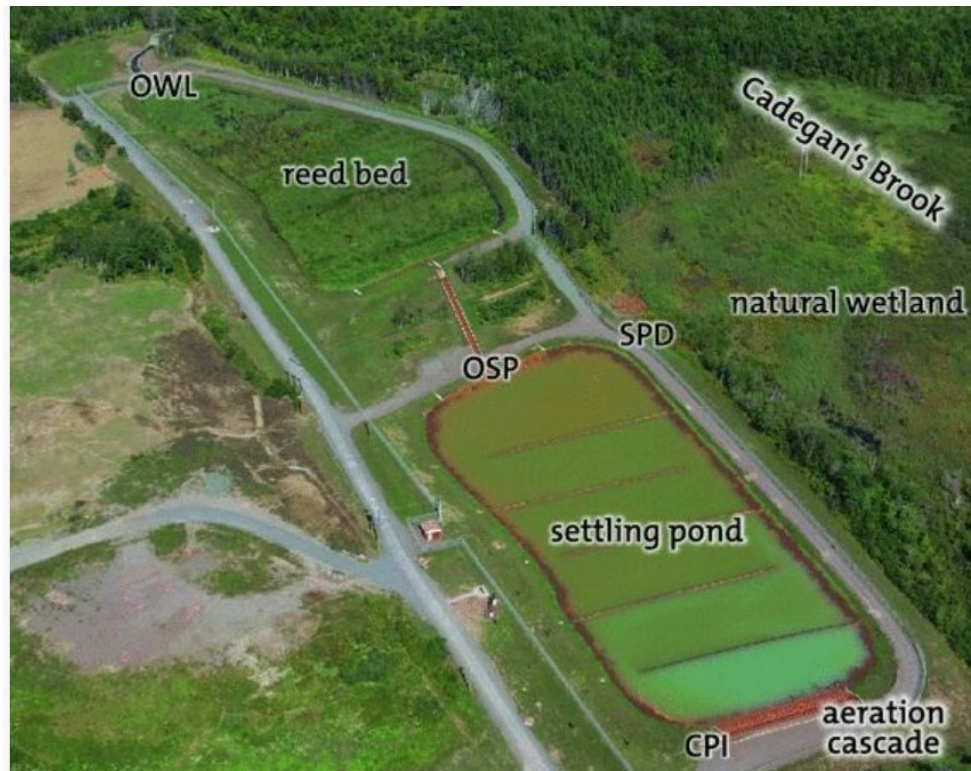
Figure 2.4 Neville St. passive treatment system in 2010 (Wolkersdorfer, 2011); OWL = outlet of constructed wetland, OSP = outlet of settling pond, SPD = settling pond discharge, CPI = cascade pond inlet.
