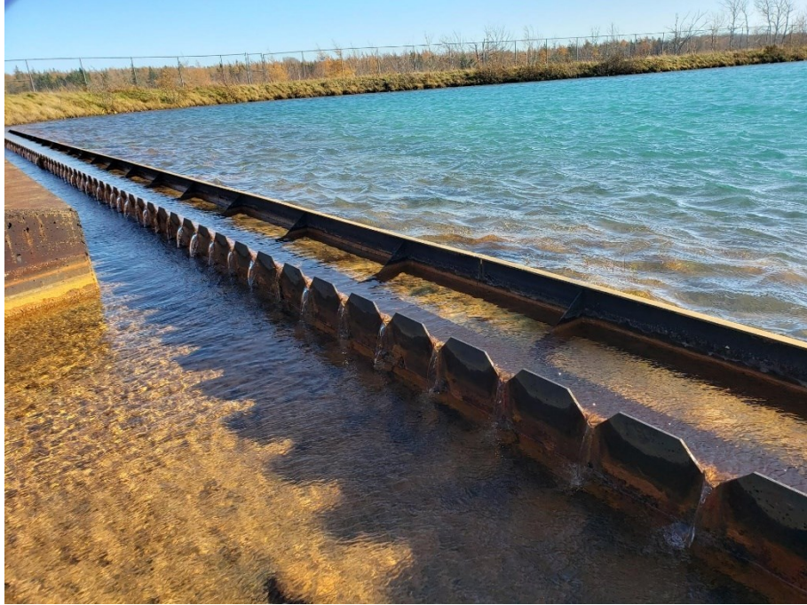
Figure A.9 Outlet structure of settling pond for System 1.
