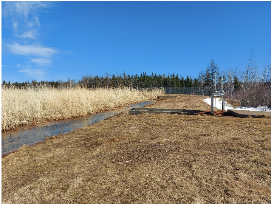
Figure A.14 Inlet of constructed wetland for System 1.
