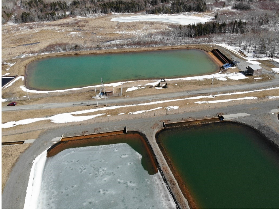
Figure A.5 Inlet and outlet structures of third settling pond for System 2 (foreground), settling pond for System 1 (middle ground), and natural wetland (background).
