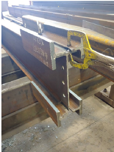
(a) T-stiffeners tack welded
