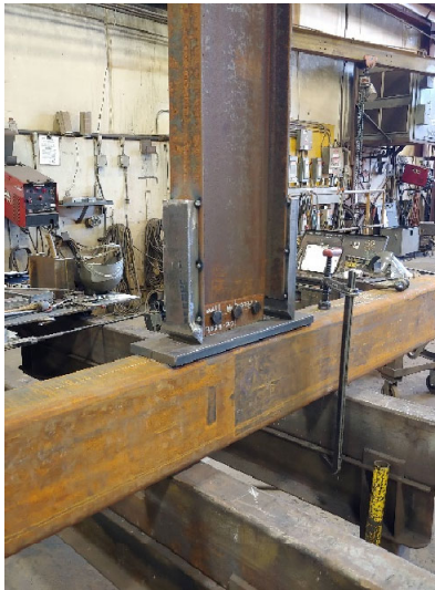
(e) flange plates tack welded
