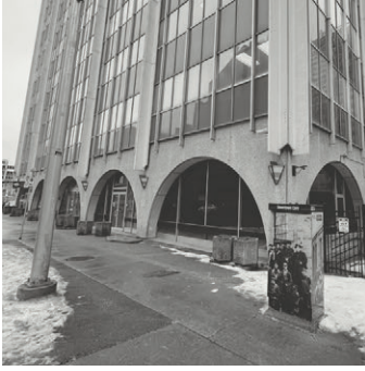
Pre-existing street front façade condition
