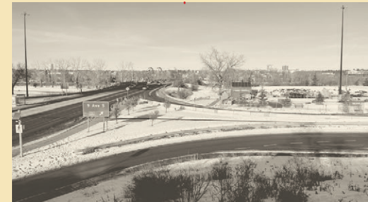
fractured connection to river valley
