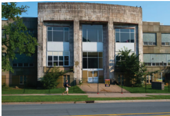
St. Patrick's high school before demolition, Halifax, NS (Taplin n.d.)
