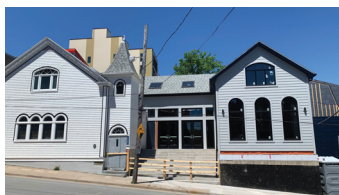
New Horizons Baptist Church undergoing renovations and an addition (NHBC 2023)
