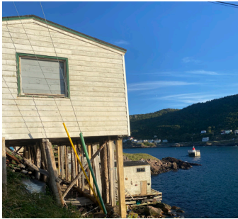
Existing Fishing Shed in the Battery, St. John's in 2019
