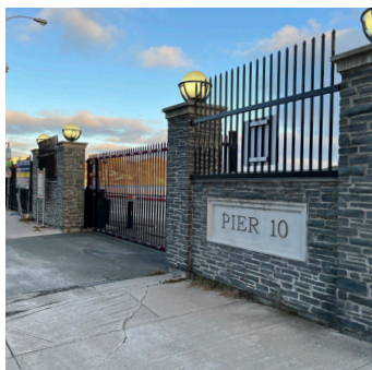
Security Fence installed by St. John’s Port Authority in 2012
