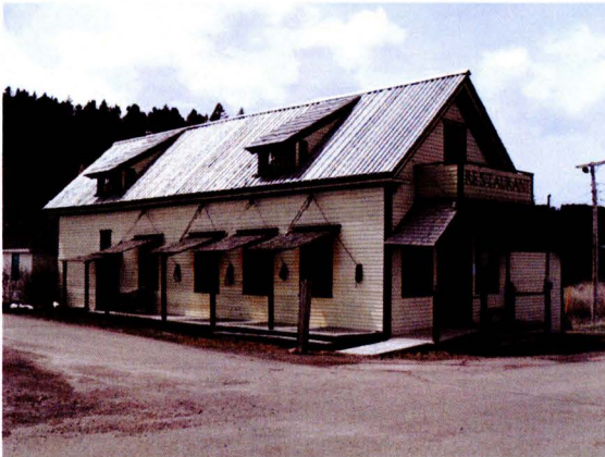
The Company store in 2007 as the Beach Cafe. The building was fitted with shutters to protect the seaward face from weathering during the off-season. During the summer they act as awnings for outdoor seating.
