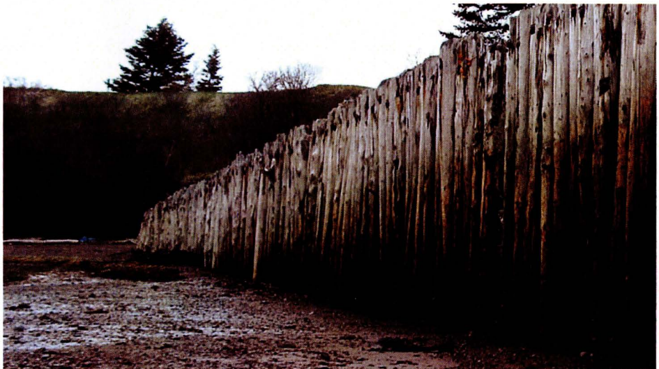
Part of the wharf in near-by Diligent River.
