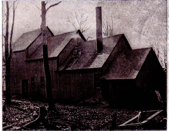
POWER AND SHAFT HOUSE NO. 1.
