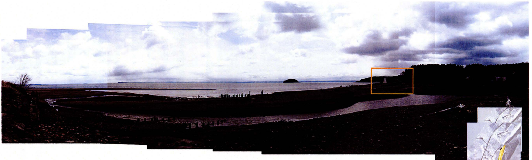
View of the lighthouse from the Shipyard node.
