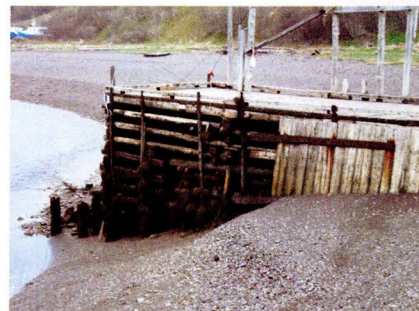
Cribbing used to moor a fishing boat in Port Greville.
