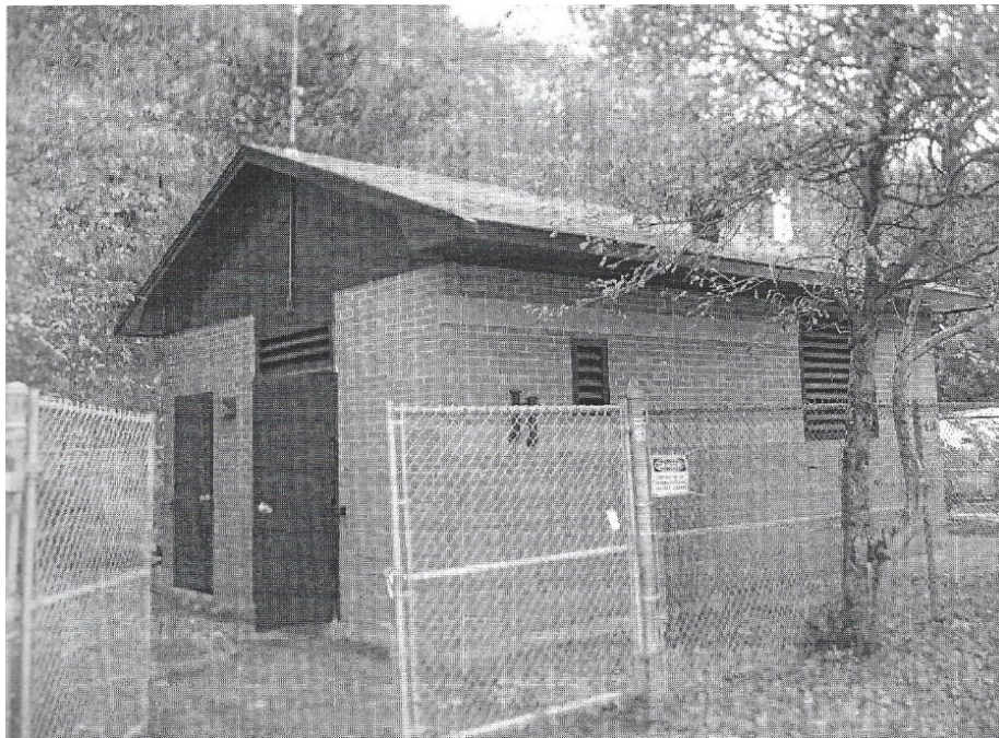
Figure 3: Example of the exterior of a medium-sized lift-station (Jean, 2006).
