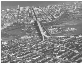
Photograph of the Burrard Street Bridge, Kitsilano Trestle Bridge, and the new Granville Street Bridge and old Granville Trestle Bridge (Matthews 1954)
