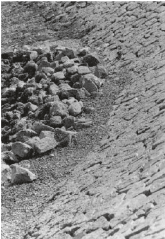
Photograph of South False Creek Seawall rockwall (Vancouver Engineering Services 1978-1983b)
