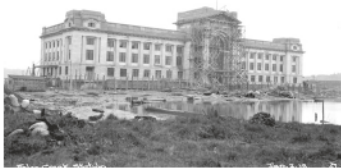
Photograph of False Creek Canadian Northern Railway station under construction (Matthews 1918)
