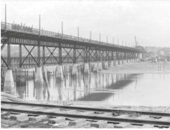
Photograph of Granville Street Bridge under construction (Matthews 1908)
