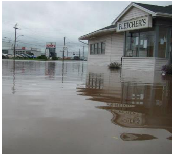
Fletcher's Restaurant in floodwater, 2012 (Scott 2012)
