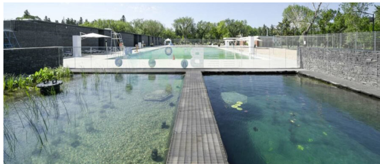
Photo of the sand filters and the swimming pool (gh3* n.d.)
