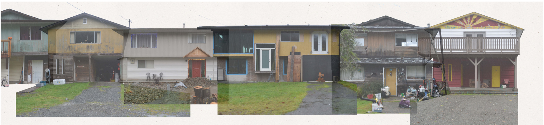
Panoramic photography of Tahsis housing with additions, ongoing maintenance, and unique aesthetic alterations to otherwise monotonous suburb housing.
