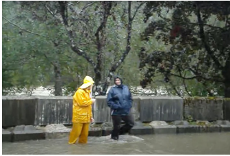
2010 floods breach the Tahsis River concrete barricades. (DeGagne 2019)
