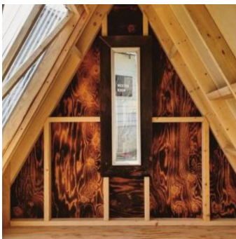
Photograph of A-frame interior framing and partial shou sugi ban finish.
