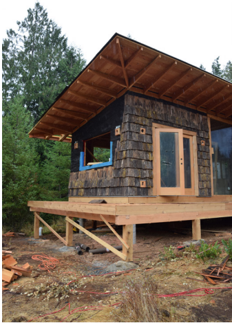
Fig. 26 A home on Gabriola Island using reclaimed cedar shingle siding.
