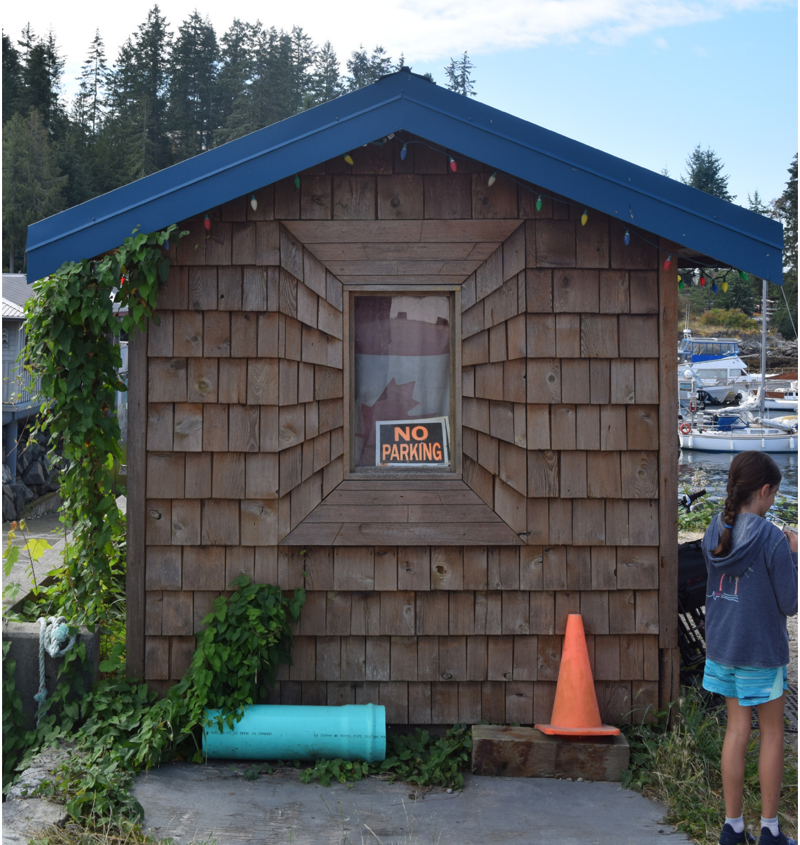
Fig. 25 A storage shed in Lund, with shingles cut into a forced perspective around the window.
