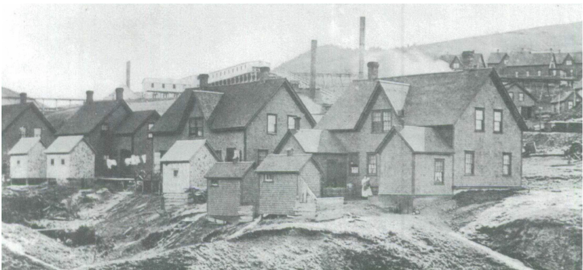
Mabou Coal Mines, Cape Breton, circa 1904. The mine was abandoned shortly after the photo was taken, and the site was stripped of all the buildings and reusable mine equipment, which was hauled to nearby Inverness. (Image and information from Muise and McIntosh 1996).
