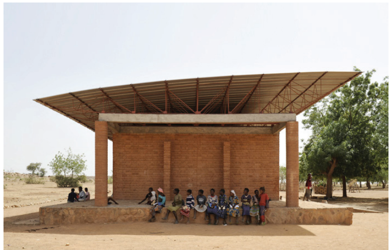
Roof of Gando Primary School (Kéré Architecture n.d.)
