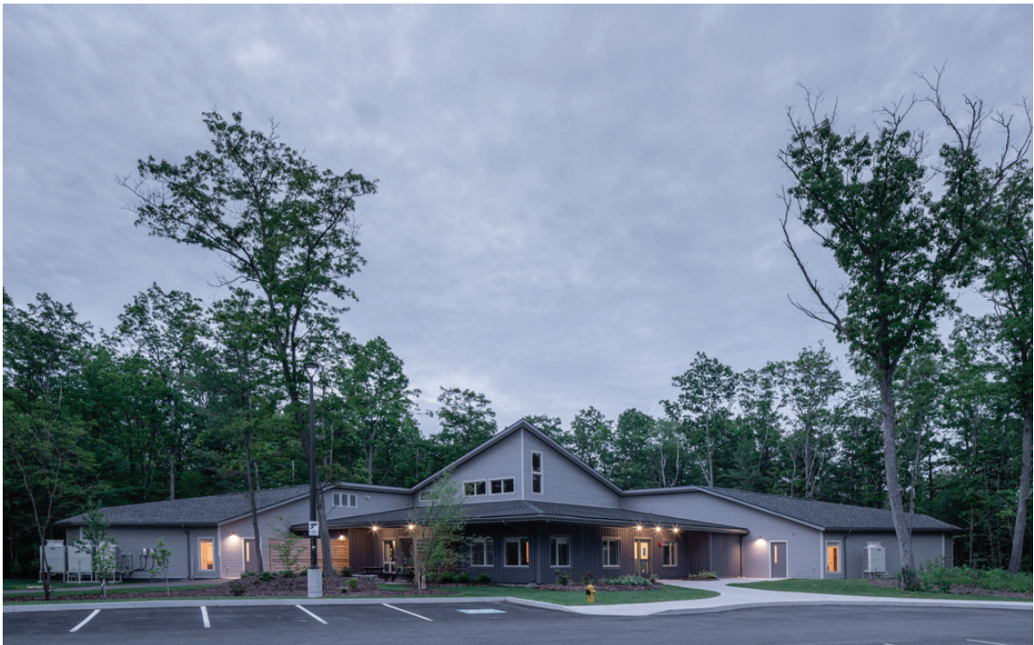
Nycum + Associates, Valley Hospice, Wolfville, Nova Scotia, 2020 (Parkinson n.d.)
