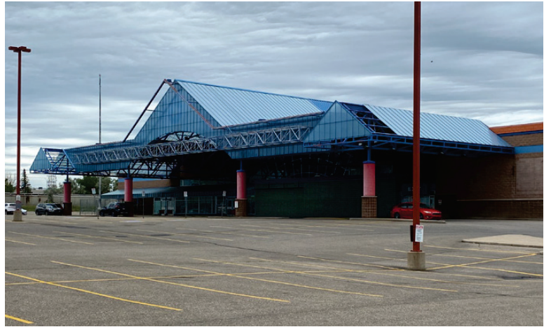
Existing building on proposed site, perspective of east side.
