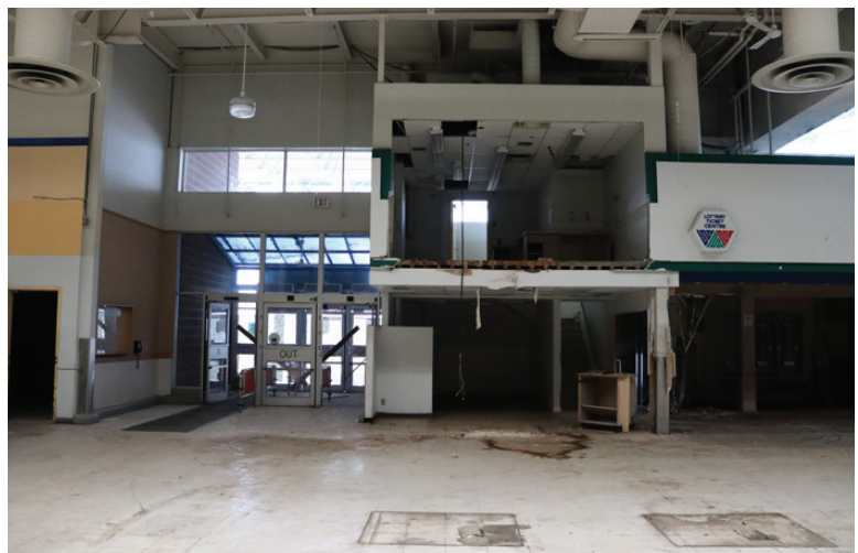
Interior image of the north-east entrance of existing building.
