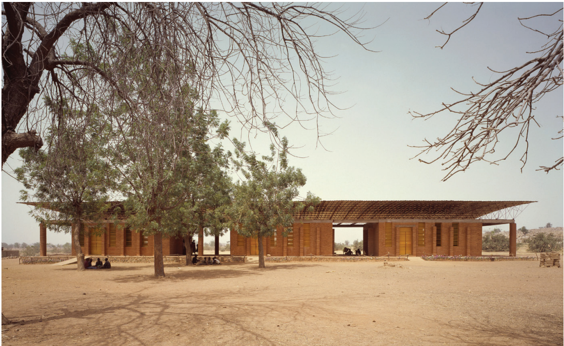
Diébédo Francis Kéré, Front of Gando Primary School, Gando, Burkina Faso, 2001 (Kéré Architecture n.d.)
