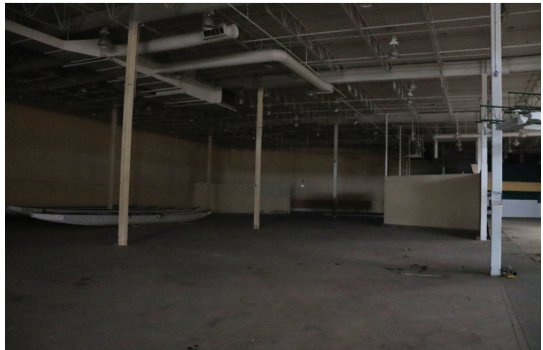
Interior image of southern most room of existing building.
