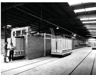
Figure 15: Tunnel kiln being loaded with bricks (Esplanade n.d.c).
