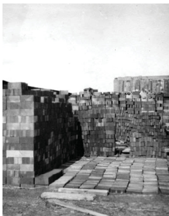
Figure 19: Red Cliff Pressed Brick stockpile on loadup platform (Esplanade n.d.c).
