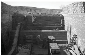
Figure 14: Assembly of temporary scove kilns (Esplanade n.d.c).
