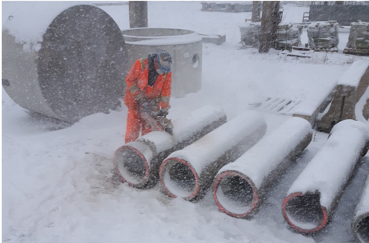
Figure 3-3:Cutting of Full-length RCP into 500mm Specimens
