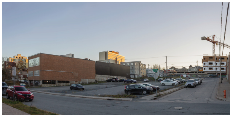
The edge of the site along Maitland Street is several meters lower, as is the typical topography along Gottingen Street.
