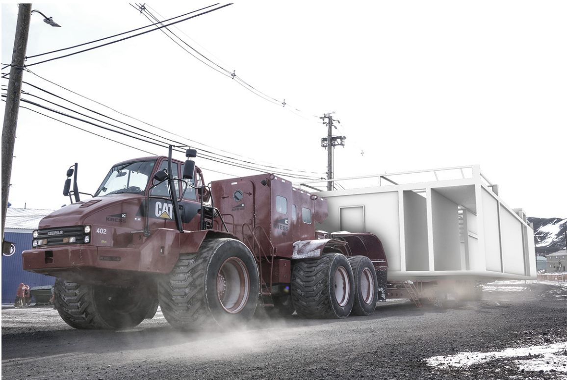
Figure 36: Moving the assemblies from the factory to the site of the habitat. Rerouting of existing utilities will be required to fully maximize the factory potential. Original photograph by Jeffery Donenfeld (USAP n.d.)
