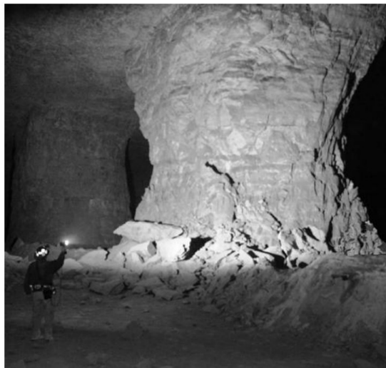
Figure 1-1: A pillar in a stone mine in Southern Appalachian area, USA (Esterhuizen et al., 2006).
