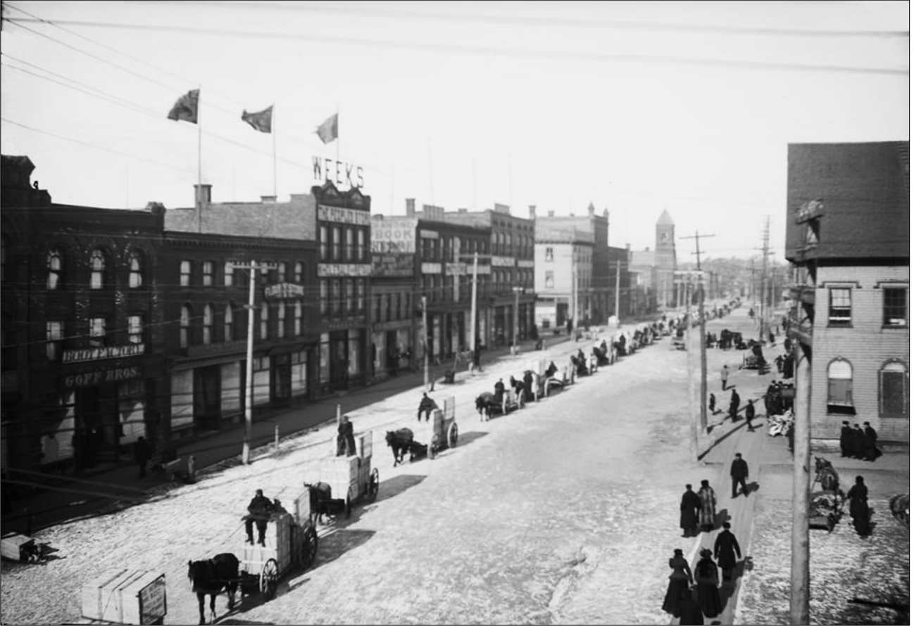
Figure 1-1: This photo of a line of delivery wagons arriving at one of Charlottetown's stores, taken by W.A Mitchell c.1900 from the corner of Queen and Richmond Streets in Charlottetown, illustrates the modern face of Maritime cities: note the wide boulevards and a crowded skyline dominated by electrical wires and store signs. Vintage Charlottetown Facebook page, November, 2012.
