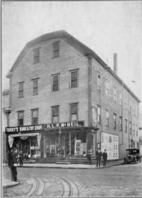
Figure 3-2: McNeil Block, 1912. Although at the time of this photo a theatre was no longer located here, this does illustrate the height and design of the building, which was common for many theatres in the Maritimes in operation in the late-nineteenth century. http://www.parl.ns.ca/industry/Business-Factory/HLPMcNeil84.jpg
