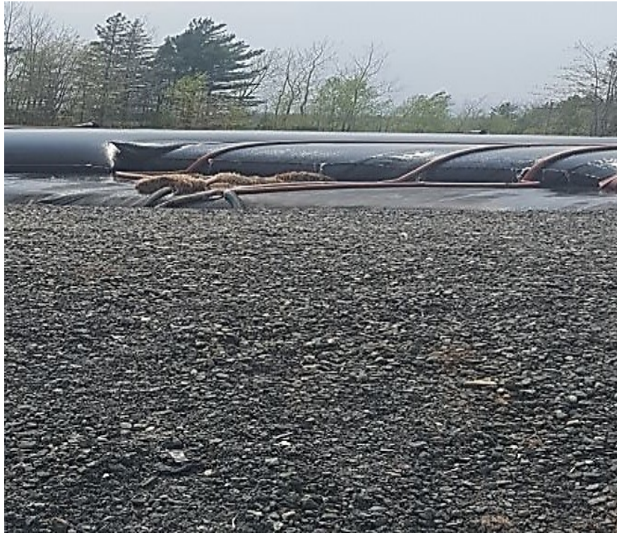
Appendix E: Geotextile tube (a filtration system) for wastewater dewatering.
