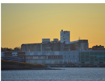
The Halifax grain elevator view from Woodside.
