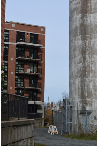
Adjacent apartments in close proximity to the grain elevator.
