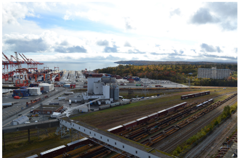
View of the harbour from the top of the grain elevator.
