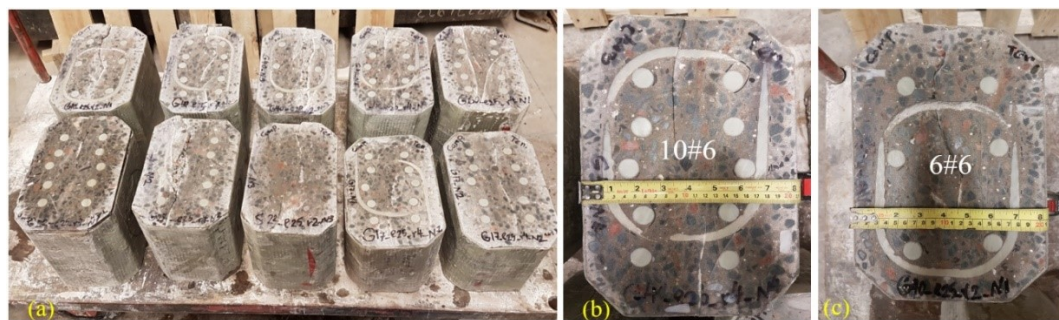
Figure 6. 3 Section cuts for rectangular GFRP-RC columns: (a) all specimen, (b) G40-N4, (c) G40-N1
