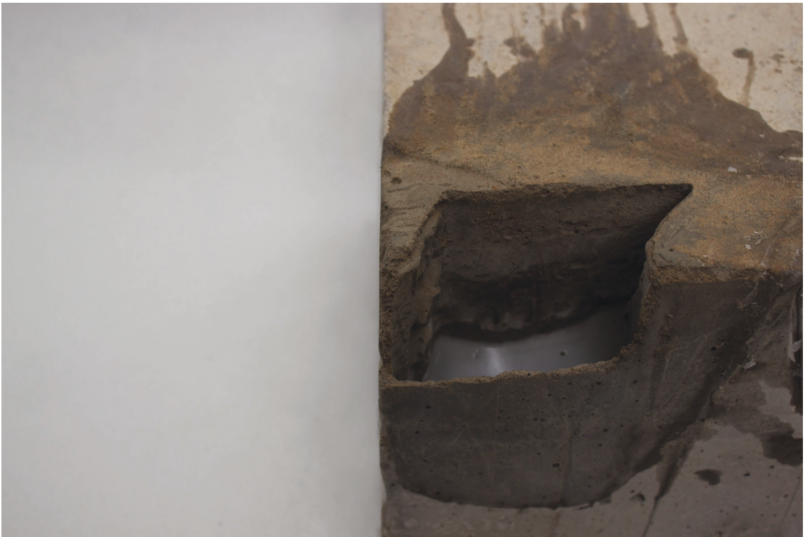
Investigation 2 - Model after wax melt out. Wax sealed the surface of the concrete, creating a finish.
