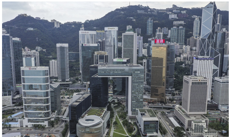
An aerial view of Central around the government headquarters.
