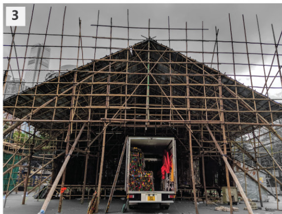
3 Bamboo canes are connected every two feet which are based on the human scale. No drawings are needed for the construction.
