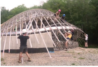
A design-build project, Cape Breton Highlands National Park Gridshell, by Coastal Studio of Dalhousie University. (Video by Coastal Studio, 2018)
