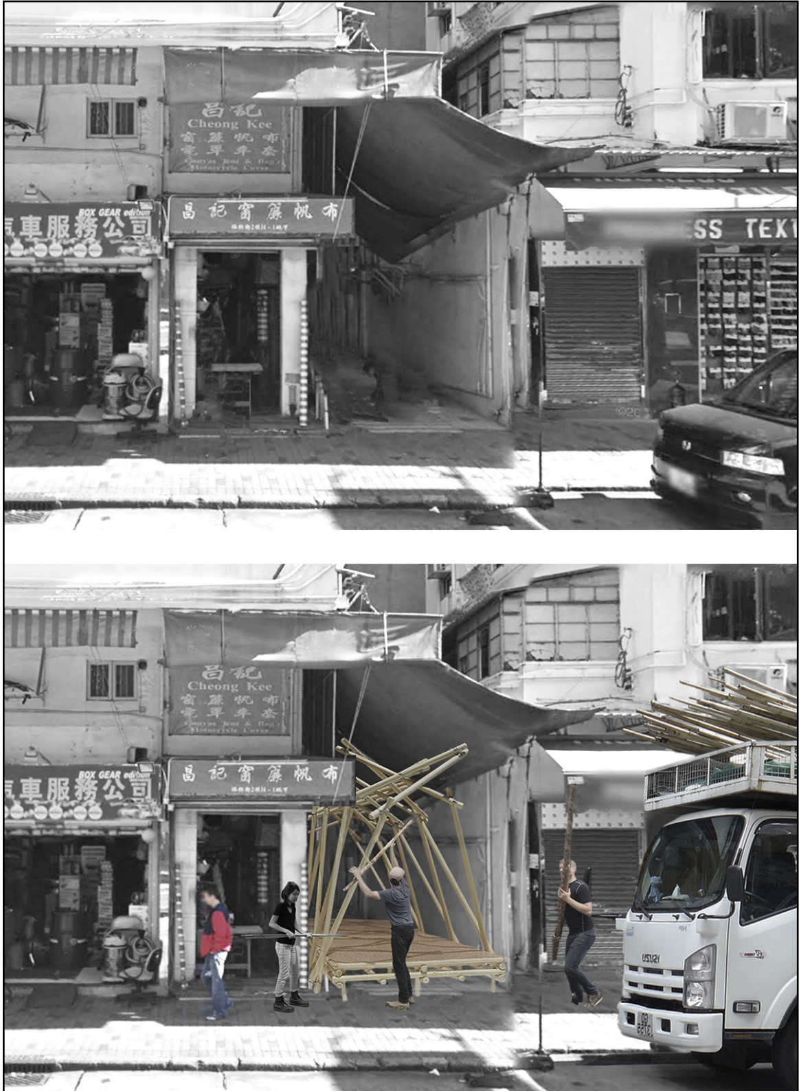
Larva is being transported on site by trucks and being constructed efficiently by bamboo scaffolders and the public who are interested in learning the techniques.
