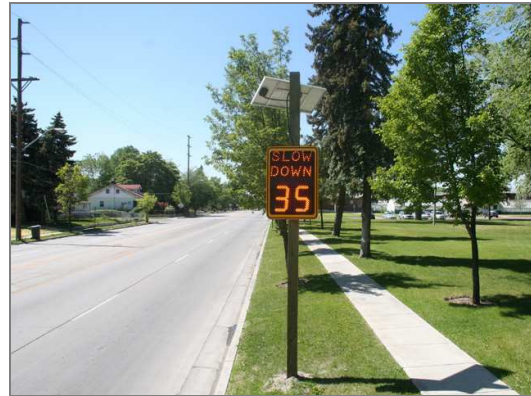
Figure 10B . View of an in-situ radar speed sign displaying the “Slow Down” variable sign. Photo by Traffic Logix.
