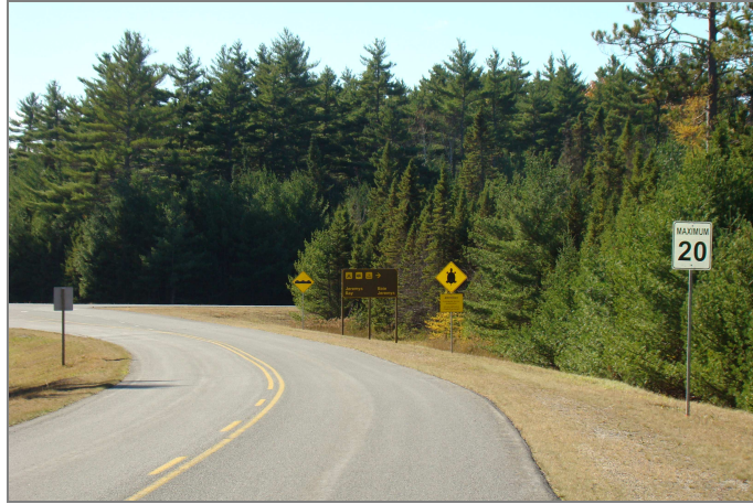
Figure 3B: View of the approach to the J-Line Road Turtle Zone management area showing cautionary turtle sign, speed reduction sign (Maximum 20), and speed bump warning sign. Photo by Heather Reed
