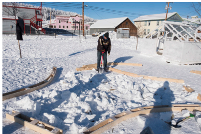
Digging out the footprint of the outdoor classroom structure.
