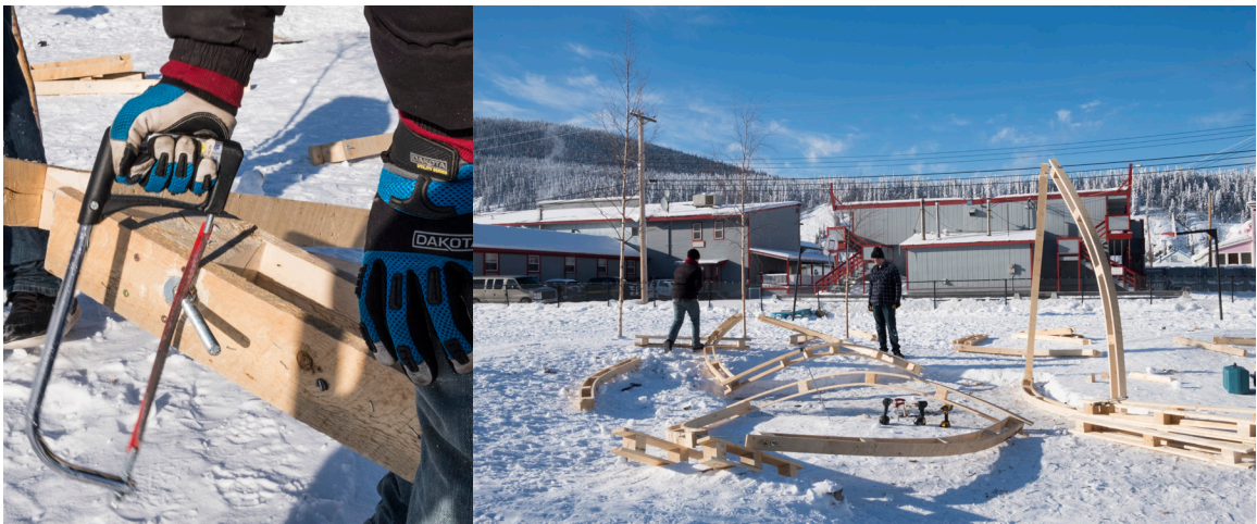
Assembling the structure on site.
