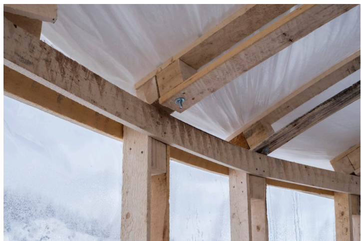
Roof to wall connection at the Riverside Gathering and Warming Pavilion.
