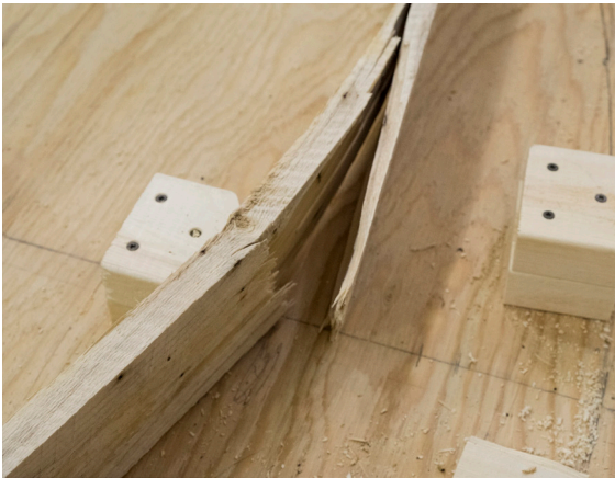
Broken 1 by 4 due to attempted bend on frozen wood.
