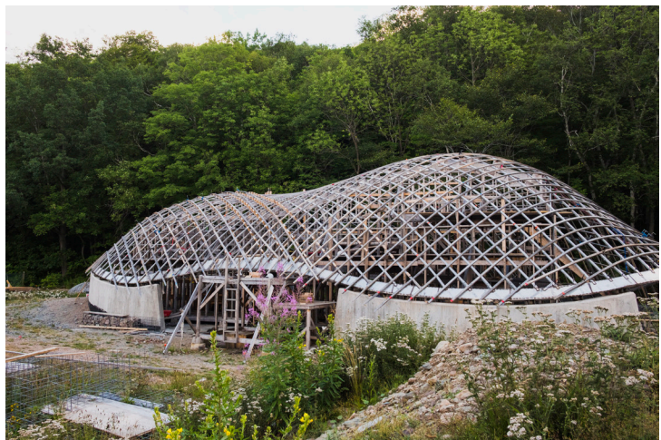
Photo of Coastal Studio Highland Gridshell under construction in August of 2018
