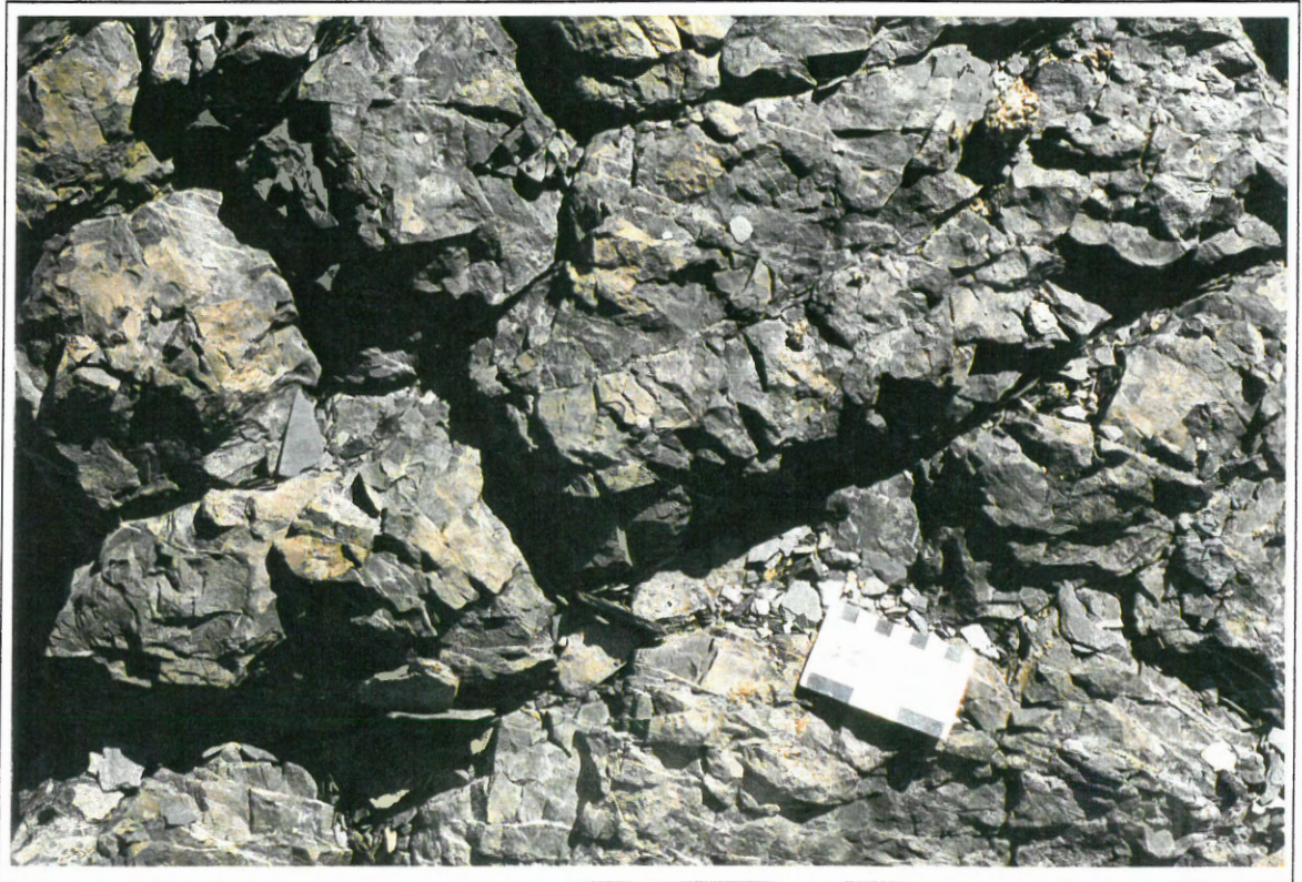
Figure 3.13 Top surface of the first tabular dolostone horizon from the coastal section at Blue Beach. Note the vertical octagonal fracturing. Thin sections reveal sediment injection structures in the uppermost surfaces.
