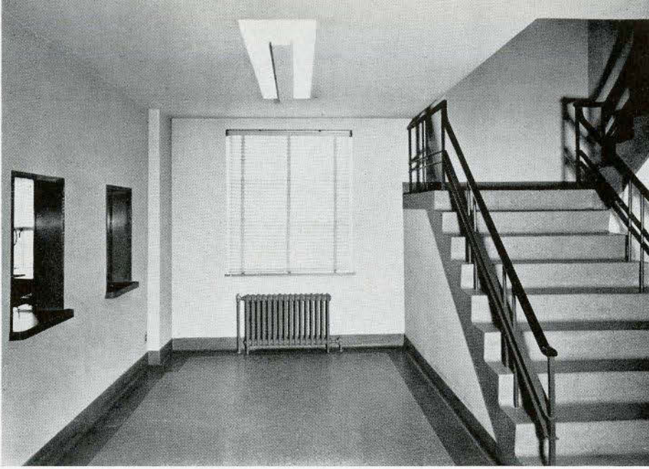
STAIR HALL, SECOND FLOOR
