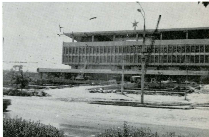
Library under construction in Tashkent.
