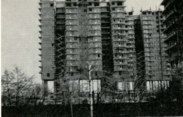
New blocks of flats under construction in Moscow from precast parts.
