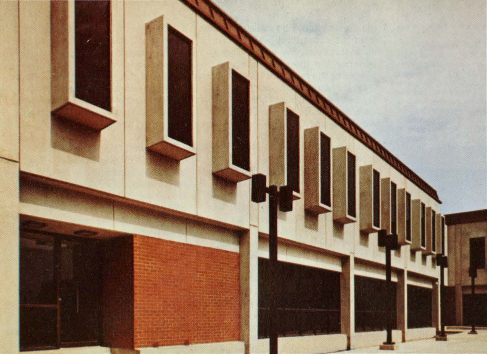
1. Effective use of decorative precast concrete panels at the Workmen's Compensation Board Building, Saint John.
