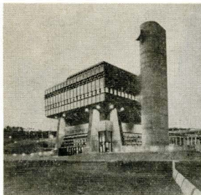
Central Control Building of the Gordon S. Shrum Generating Station on the Peace River in northern BC. Rhone and Iredale, Bogue Babicki and International Power and Engineering Consultants
