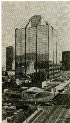
Westcoast Transmission building, Vancouver, the first continuous cable-suspended building in North America. Bogue Babicki & Assoc., structural engineers, Rhone and Iredale, project architects
