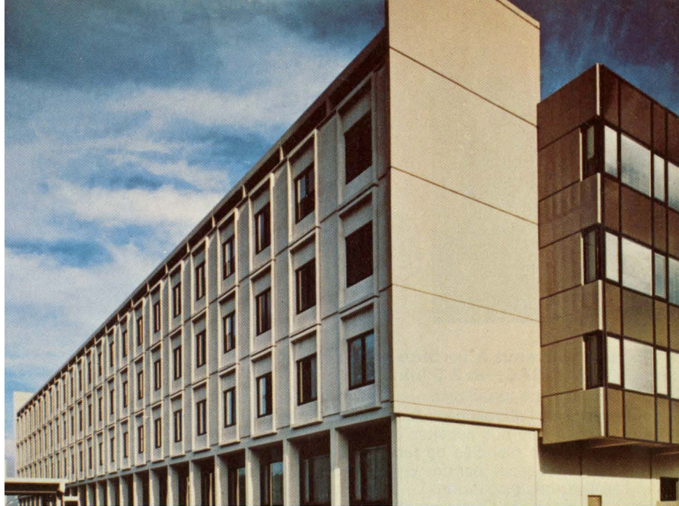
5. Acute Treatment Building, Kelowna General Hospital, B.C., is built in concrete with precast concrete exterior walls.
