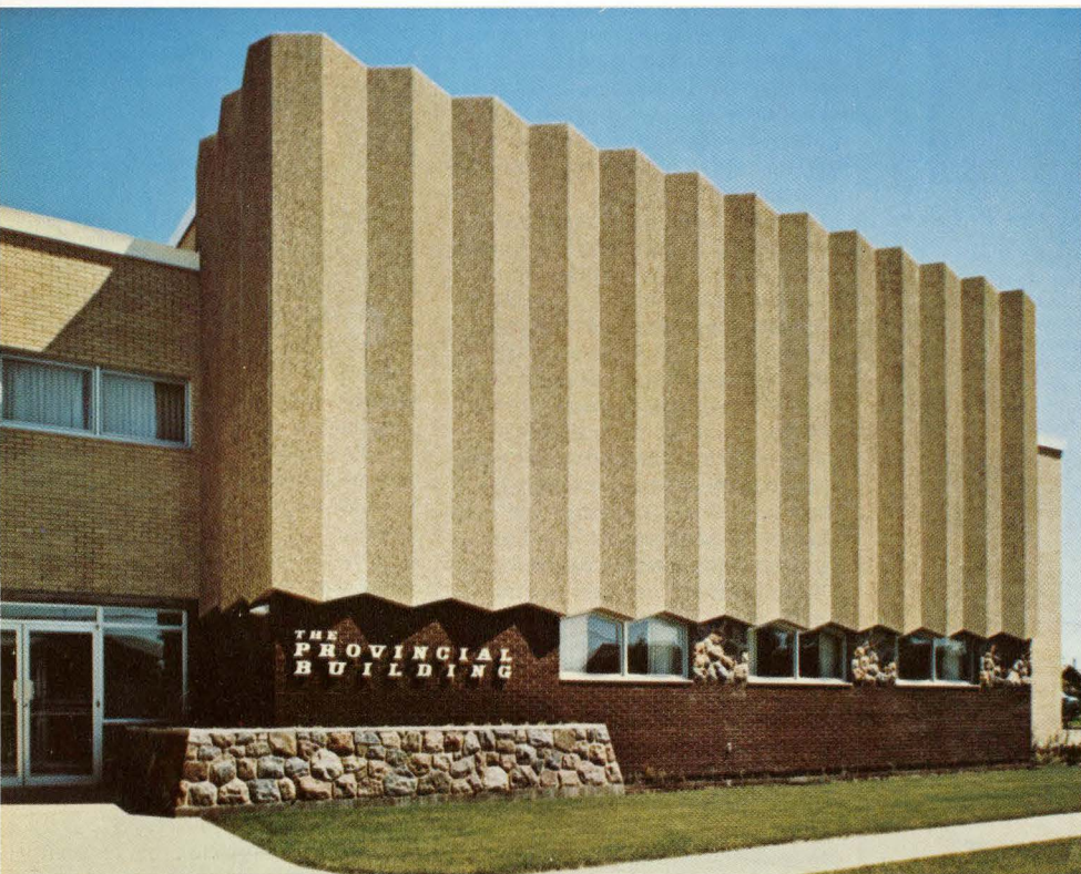
2. Exposed aggregate precast panels enhance the beauty of The Provincial Building, Melville, Sask.
