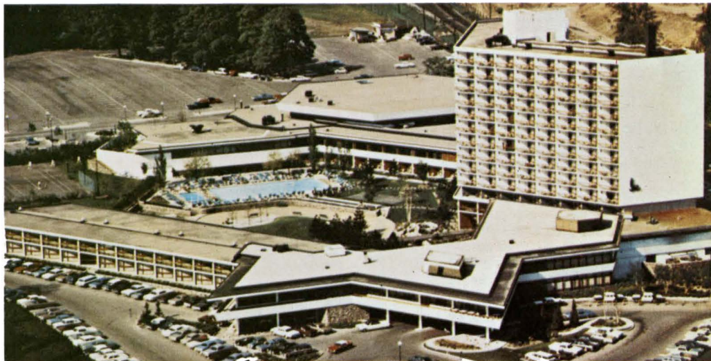
The new high-rise section of the Inn on the Park, Toronto, Ont., built with lightweight aggregate concrete.
