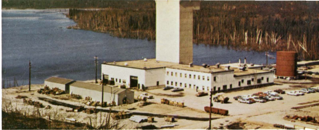
The graceful concrete No. 3 Headframe of International Nickel Company at Thompson, Man.
