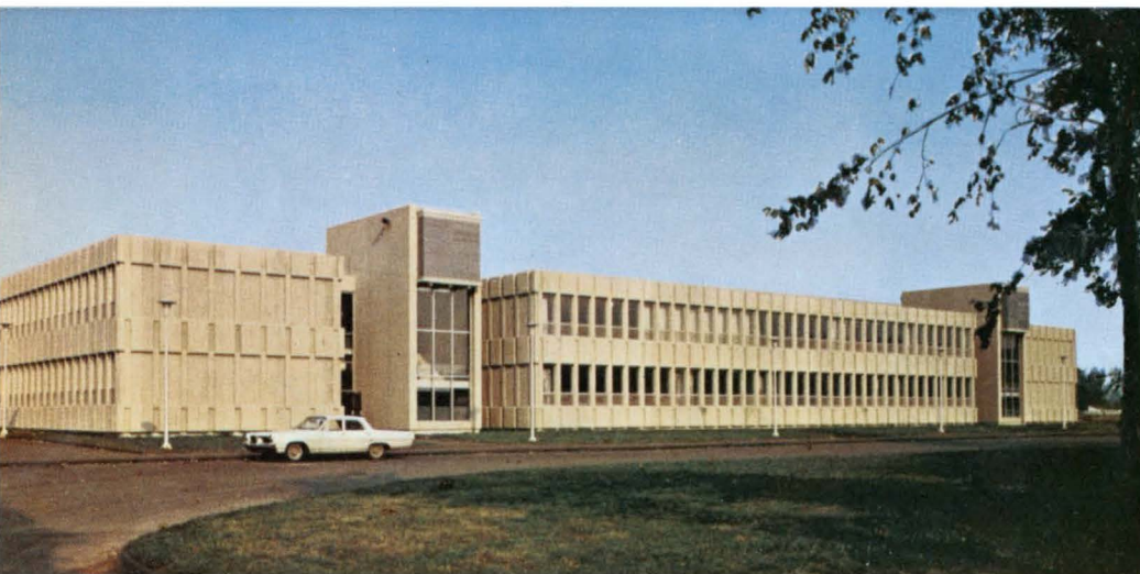
The Regional Polyvalent School, Huntingdon, Que., was built of concrete for economy and fire safety.
