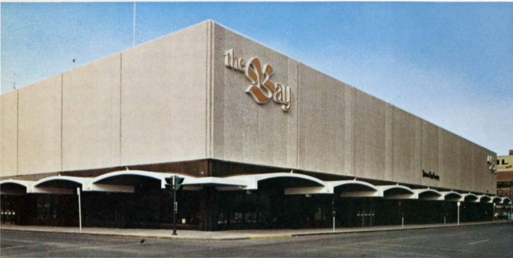
Precast concrete panels lend elegance to the Hudson's Bay Company department store at Regina, Sask.
