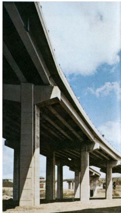
The all-concrete elevated roads of the north
