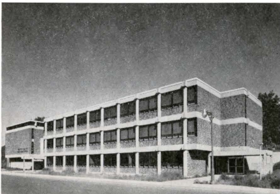
Beth Jacob School, Montreal. Arch: Schrier & Kessler. Genl. Contr: Montclair Construction Co. Ltd. Masonry Contr: A. Croteau & Fils Inc. Concrete & Precast Concrete Members: Francon Ltd.
