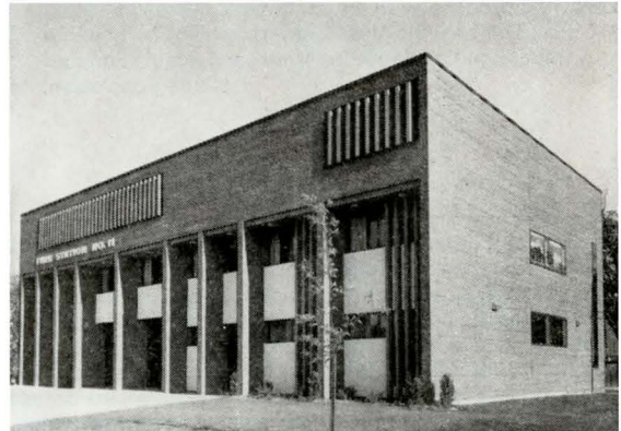
Fire & Welfare Building, Toronto. Owned, designed & built by: City of Toronto. Masonry Contr: D.M.S. Contractors Limited. "Canada" Masonry Cement Supplied by: Community Building Supplies Ltd.
