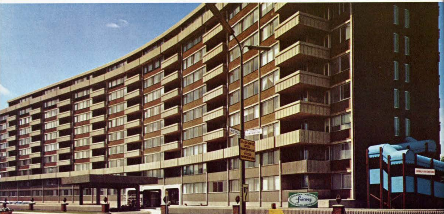
1 (Top left) Avord Tower, Regina, Sask. 2 (Top right) Victoria Park Apartment Building, Halifax, N.S. 3 (Bottom) Fairway House, Cote St. Luc, Que.
