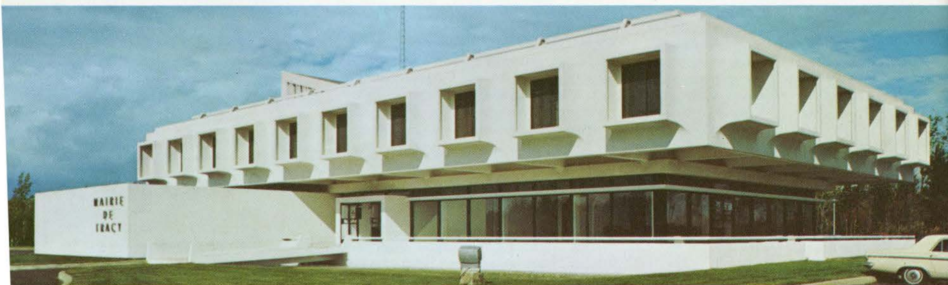
4. Imaginatively designed concrete panels provide unusual beauty and flawless uniformity for the City Hall, Tracy, Que.
