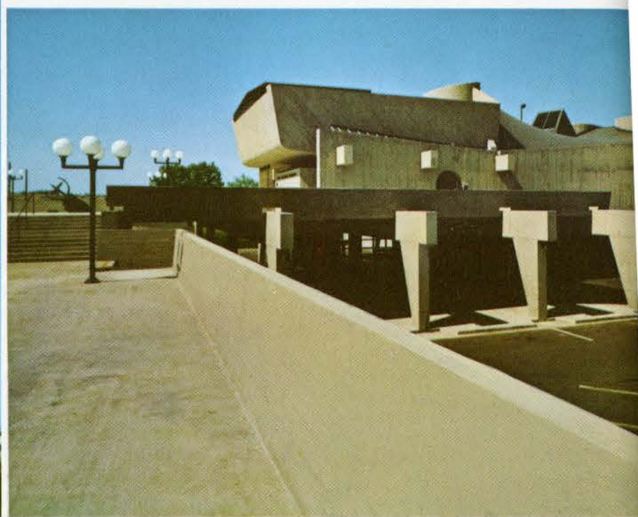
3. Bold concrete design for the Centennial Planetarium, Calgary, Alta.
