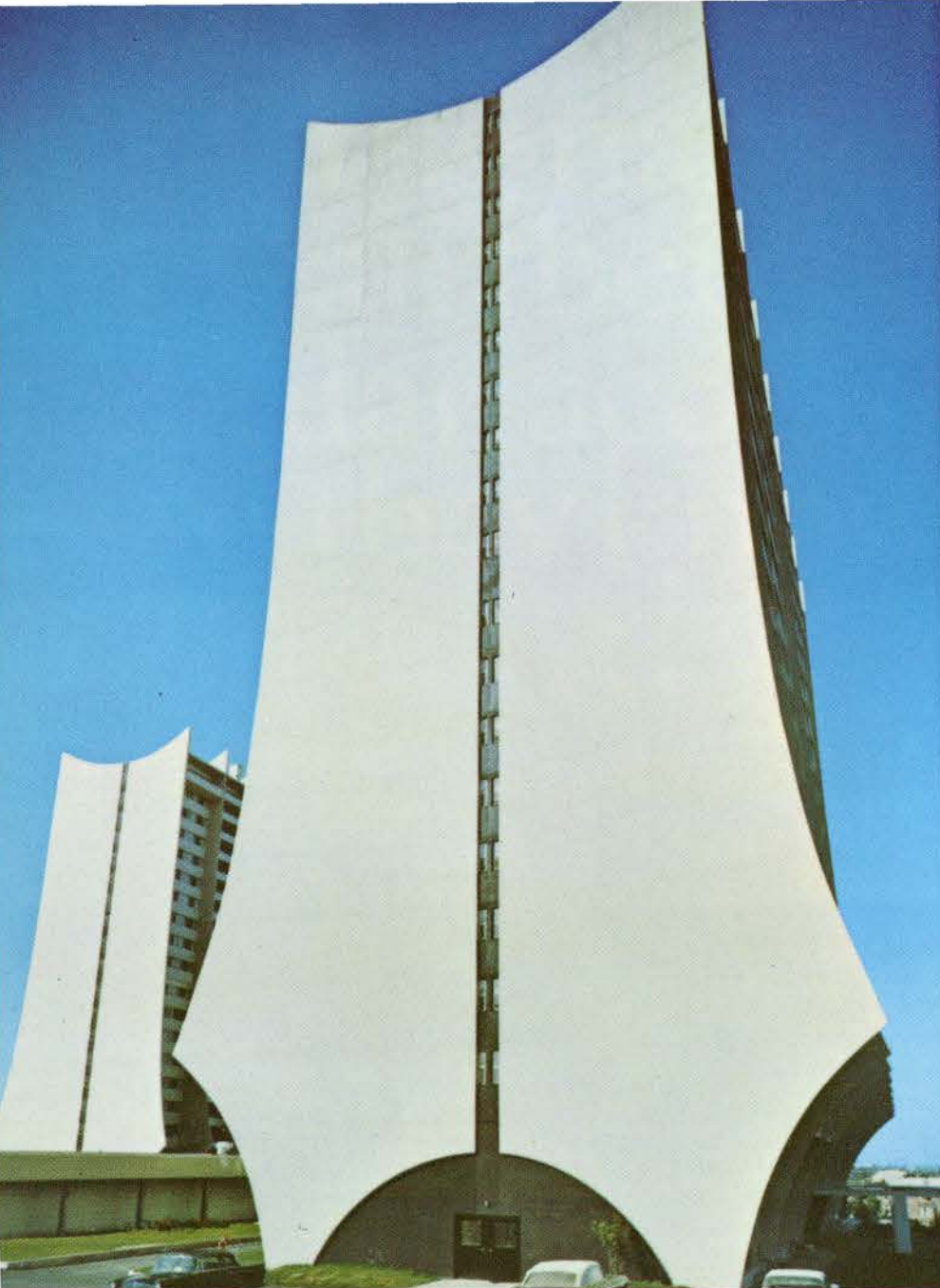
1. The spectacular North York Exbury Towers, Toronto, Ont.
