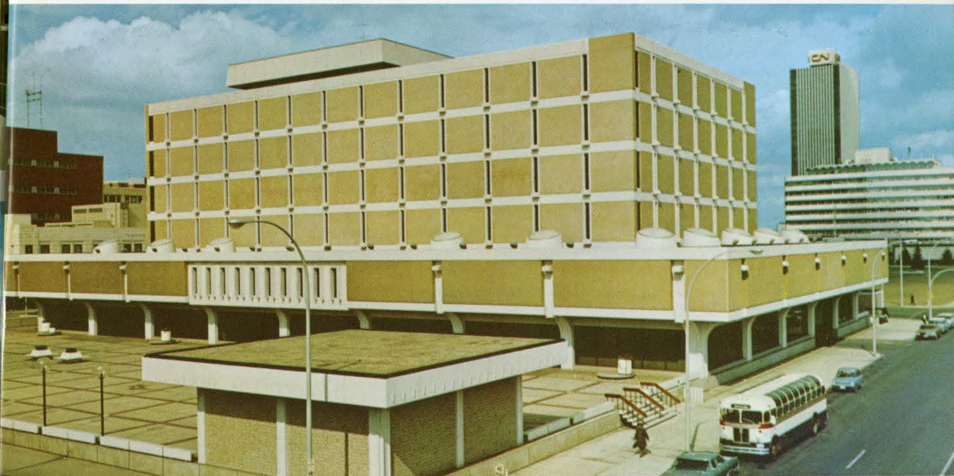
7. The Edmonton Centennial Library, a fine example of precast concrete construction. The CN Tower can be seen in background.
