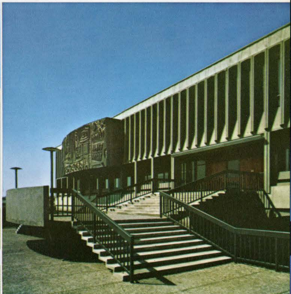
8. The precast concrete Bishop Grandin Academic & Vocational High School, Calgary, Alta.
