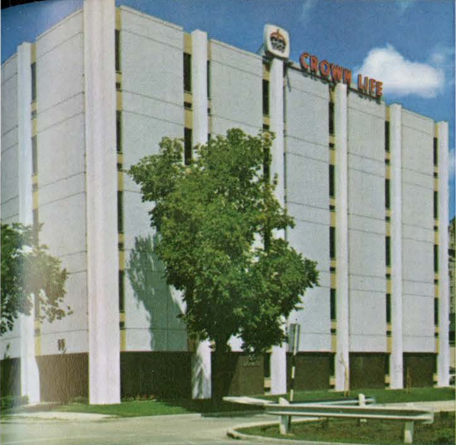
7. The Oldfield, Kirby & Gardner Building, Winnipeg, Man., an all-concrete structure.
