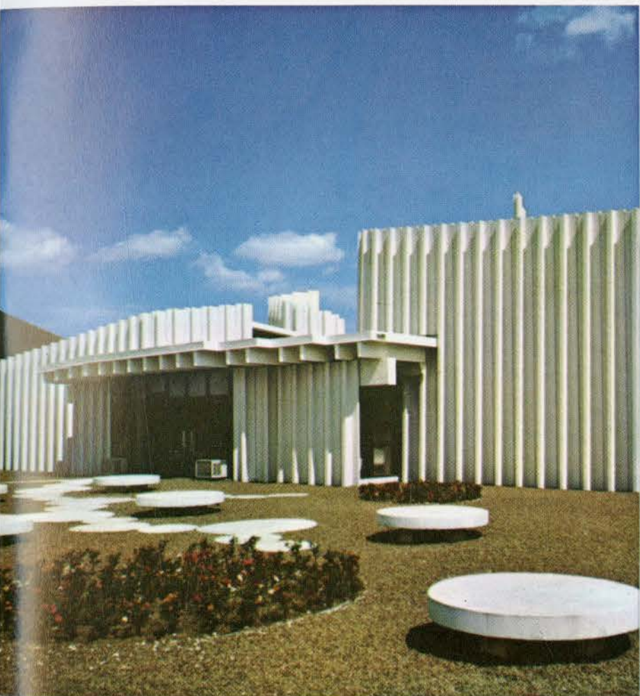
7. The all-precast concrete Man and Music Pavilion at Expo 67 can be dismantled.
