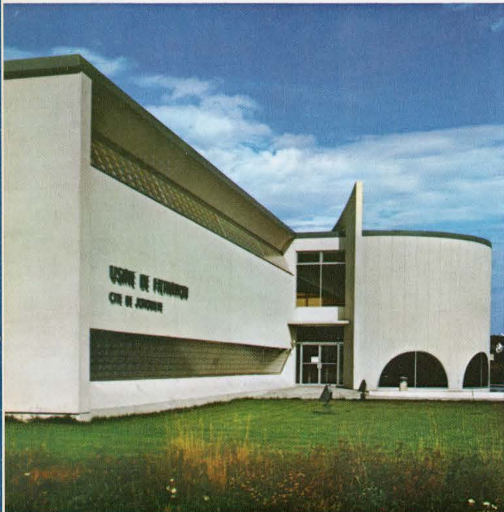
5. Cast-in-place concrete molded the shape of this Filtration Plant at Jonquière, Que.
