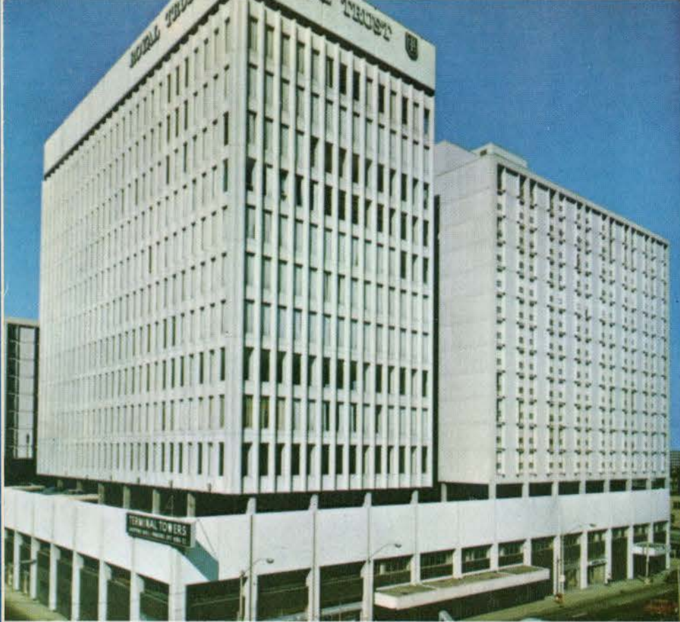
1. The Terminal Towers, Hamilton, Ont., features precast concrete panels.
