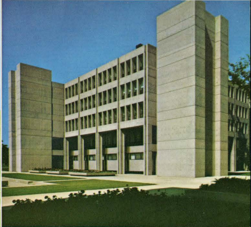
4. Exposed concrete walls for the Health & Welfare Building, Charlottetown, P.E.I.
