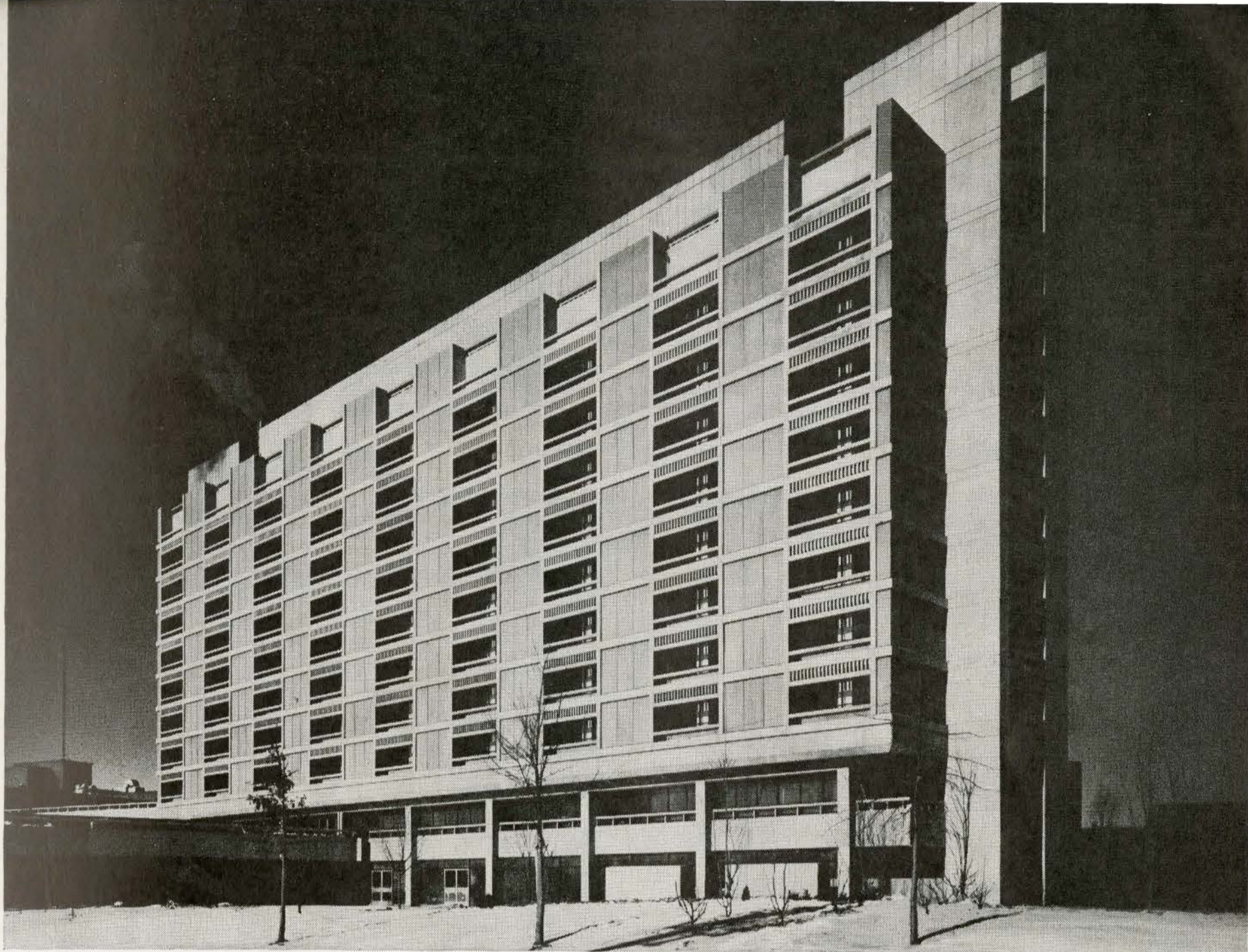
Jewish Home for the Aged, Toronto • Architect: Marani, Rounthwaite & Dick • Associate Architect: Jerome Markson • Contractor: Redfern Construction
