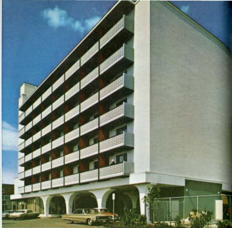
2. A variety of concrete masonry units for the Riviera Motor Hotel, Edmonton, Alta.
