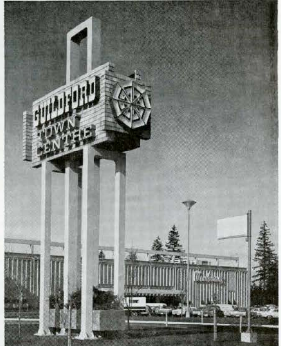
Guildford Town Centre, Surrey, B. C. Architect: Frank Donaldson. Consulting Engineer: Phillips, Barratt & Partners, Vancouver. Contractor: Laing Construction & Equipment Ltd., New Westminster, B.C.
