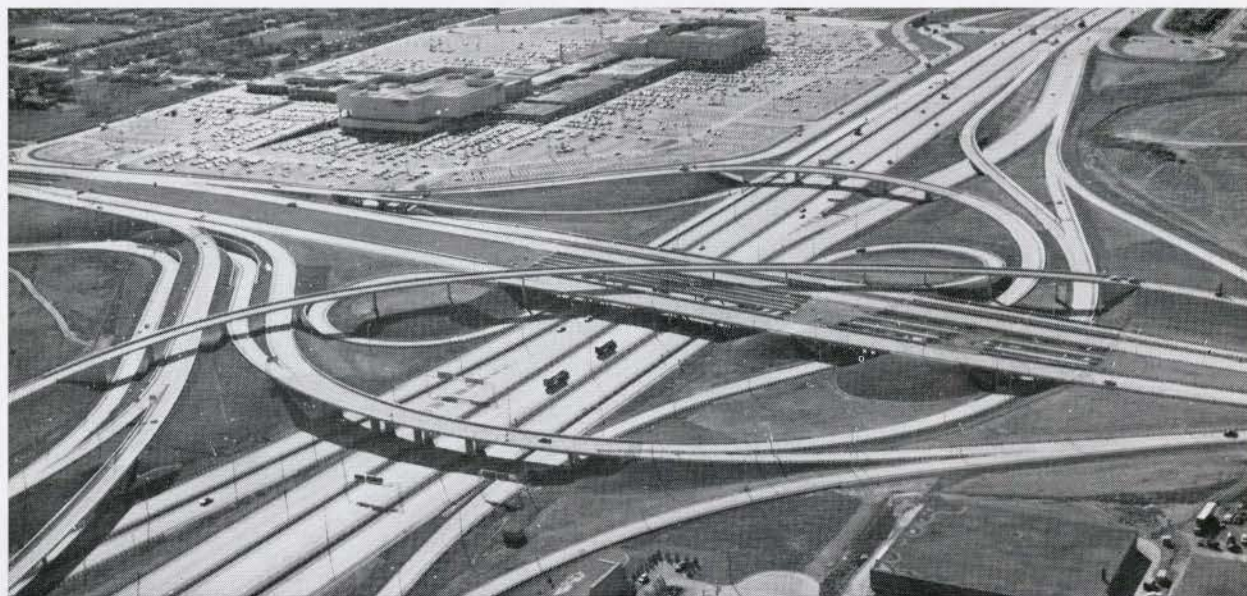
Photo: Department of Highways, Ontario.
