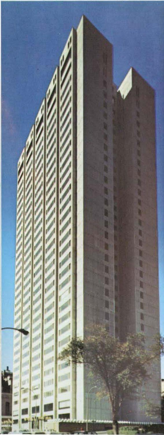
1 Port Royal Apartment Building, Montreal, Que.
