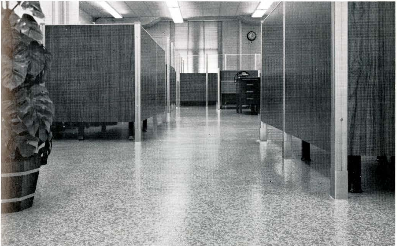
Below, new Tessera Corlon floor installed over old linoleum by time-saving Perimiflor System.
