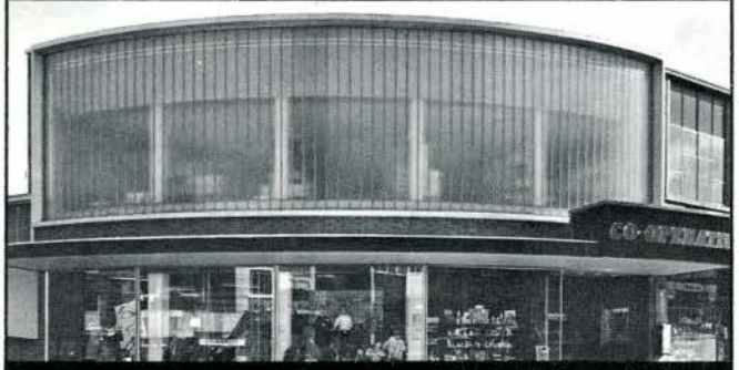
The curved elevation on the second story of this building is glazed with Profilit Glass.
