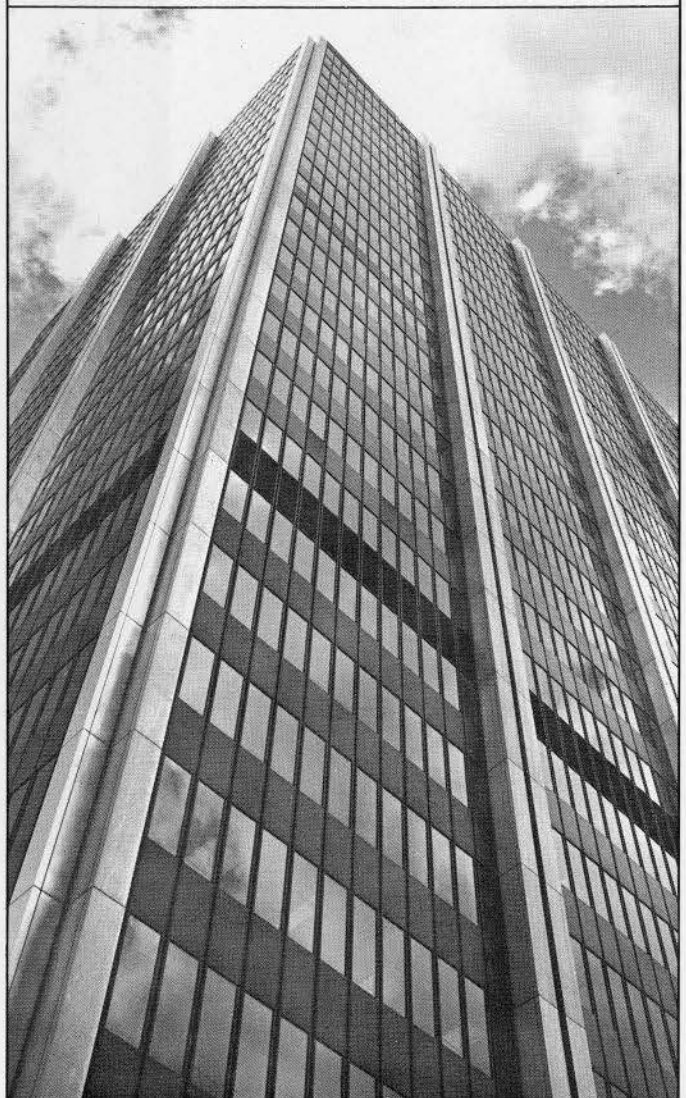
The new Richmond-Adelaide Centre, Toronto. A beautiful example of a complete curtain wall project.
