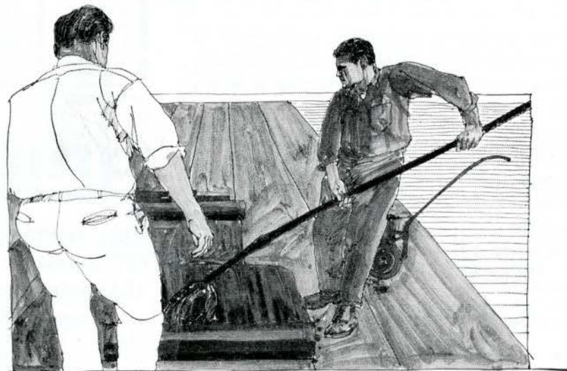
Felt being mopped over factory-coated base sheet. Hot asphalt does not contact Roofmate FR.
