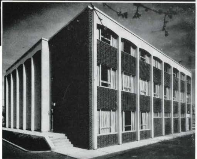
MAGISTRATES COURT BUILDING, Willowdale, Ont. ARCHITECT: Sproatt and Rolph GEN. CONTR.: Stowe and Gould Ltd. PRECAST PANELS BY: Pre-Con Murray Ltd.
